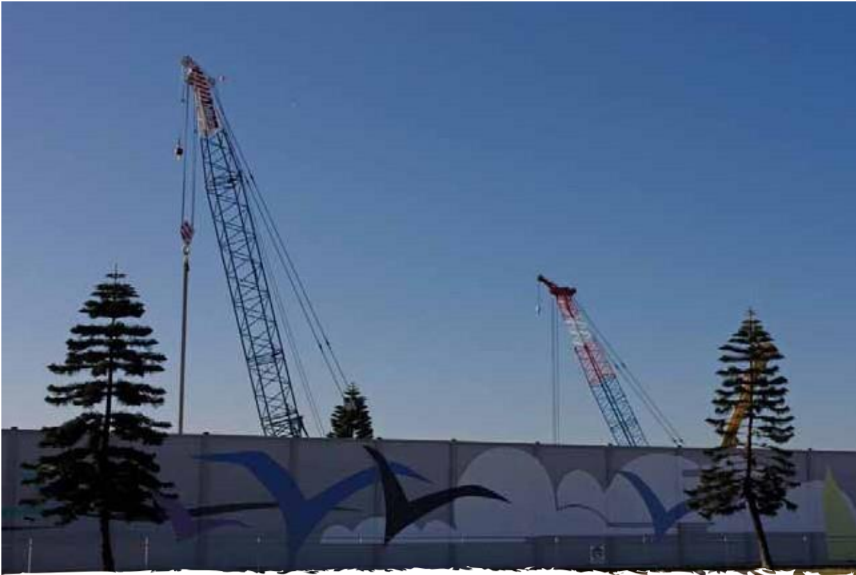
Temporary noise barriers around a pipeline worksite (DECC)
