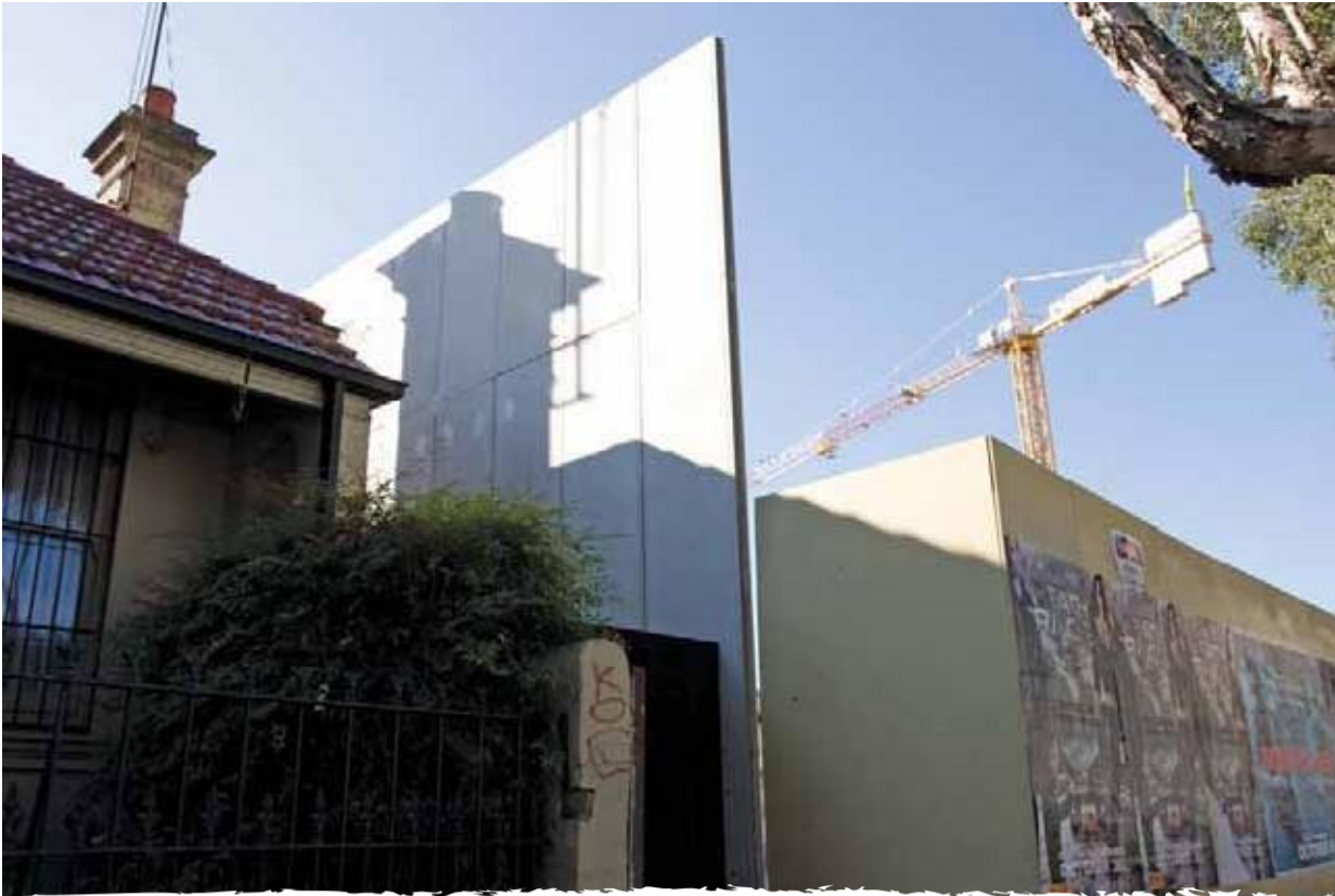
A temporary noise barrier between the worksite and a neighbour (DECC)
