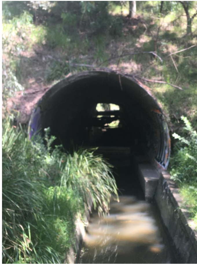
Image #3: Storm Water Tunnel East
