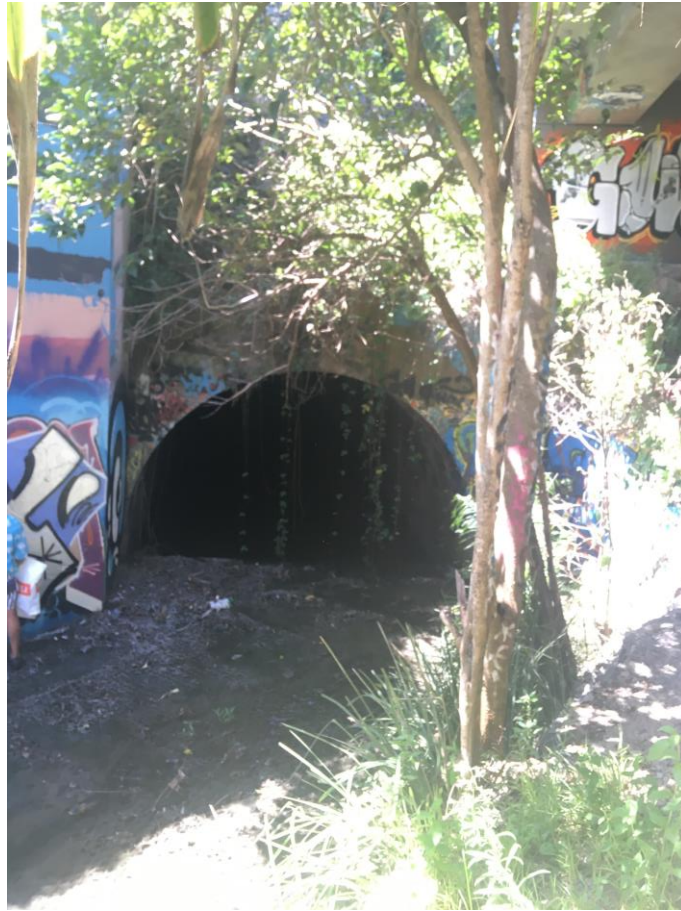
Image #4: Storm Water Tunnel West
