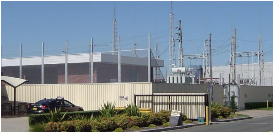
Endeavour Energy's Seven Hills Zone Substation is an 'outdoor' design. Note height of fencing due to adjacent 'climb point' created by the seating and awning. Source: Google Maps Street View.
