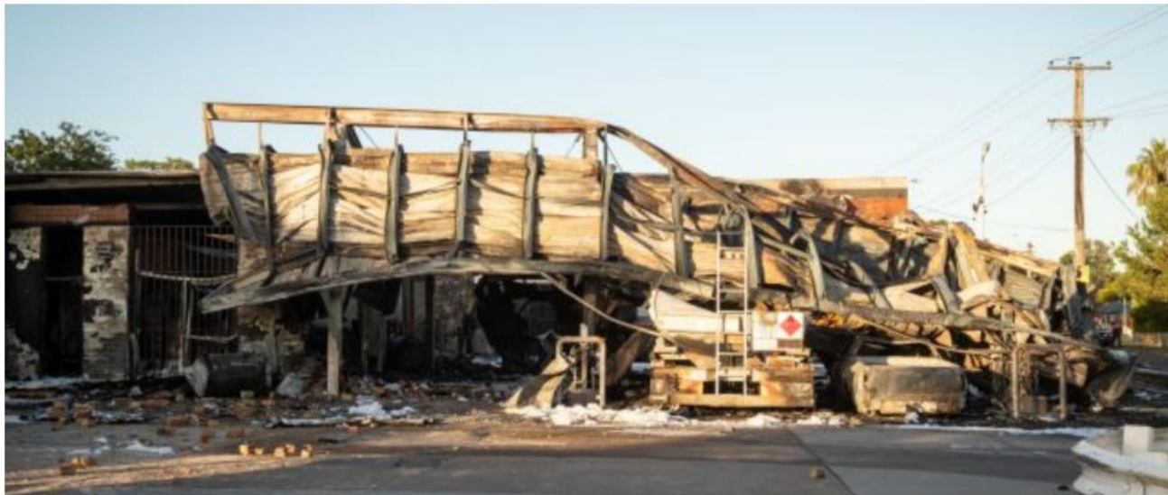
Figure 4: Service Station Facility Following Fire
