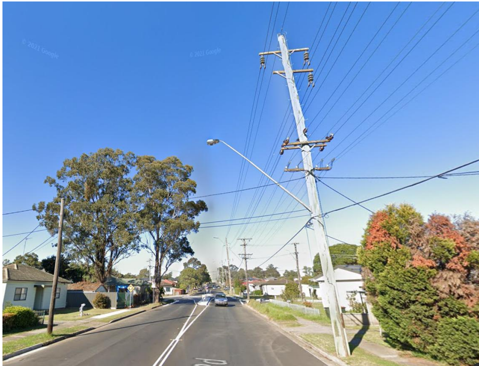
Overhead powerlines with high voltage, low voltage and service connections at different levels on the poles. This example is in Marayong NSW part of Endeavour Energy's franchise / network area. Source: Google Maps Street View.
