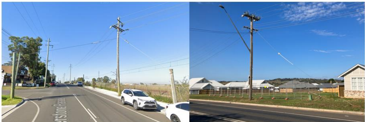
Stay poles at Riverstone Source: Google Maps Street View. Ground stay at Menangle which with the urban residential subdivision may need to be replaced with a bollard pole.
