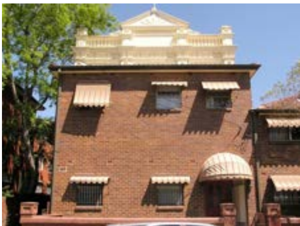
Figure 17. The elaborate Victorian terrace on this property in Cambridge Street has been obscured by this highly unsympathetic and aesthetically ungainly proportioned extension towards the street. It is not known whether the original facade was removed or whether it still exists within the building.
