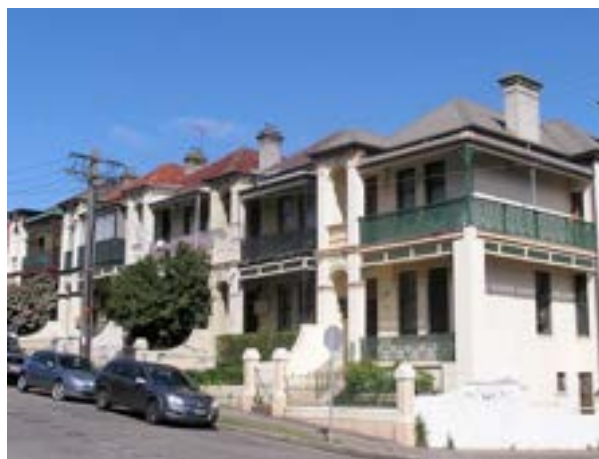
Figure 10. This imposing row of town houses rises up Cavendish Street from the low point where it meets Merchant Street. Their consistent form and setback contributes to the strongly patterned streetscapes near this intersection.
