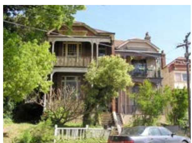
Figure 53. Trafalgar Street terraces.
