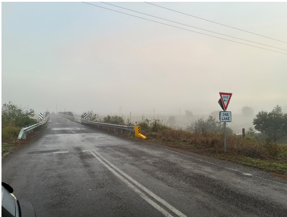
Figure: Elderslie Bridge during foggy conditions with poor visibility conditions
