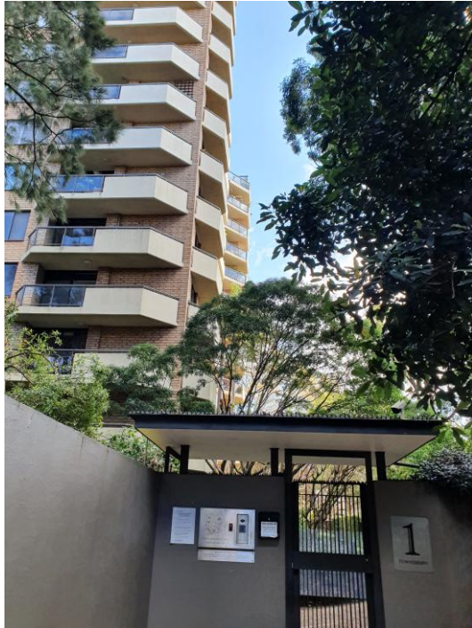
1 Tewkesbury Avenue, showing glazed balconies
