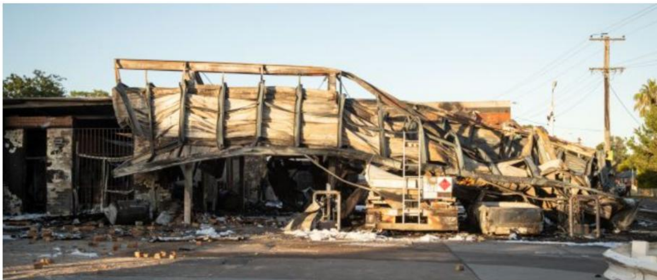
Figure 4: Service Station Facility Following Fire
