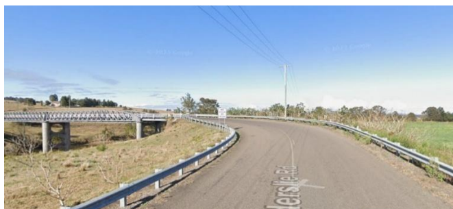
Figure 1 Elderslie Bridge Approach Southbound
