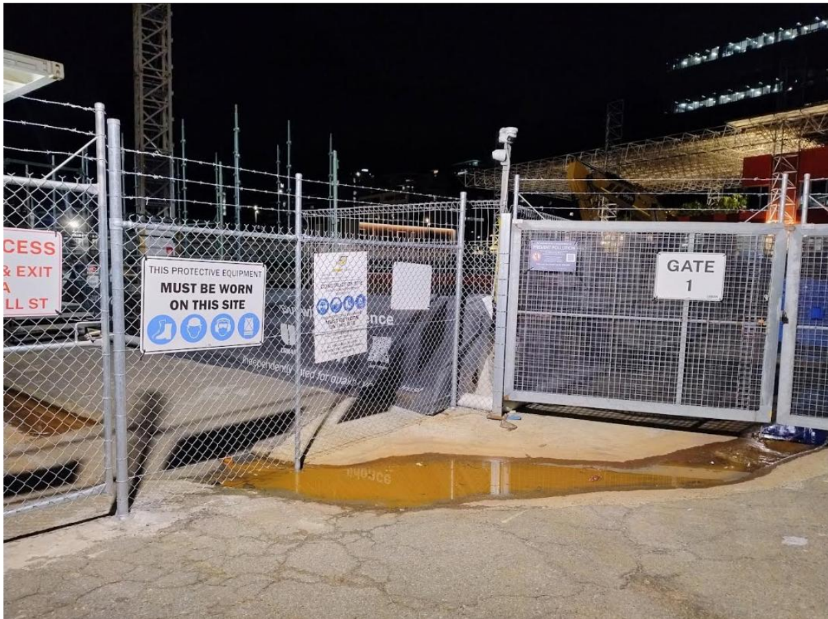
Figure 1 (Author's Own) June 2026. Orange-brown staining of ground and site runoff
