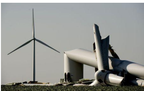
Turbines can fail catastrophically
