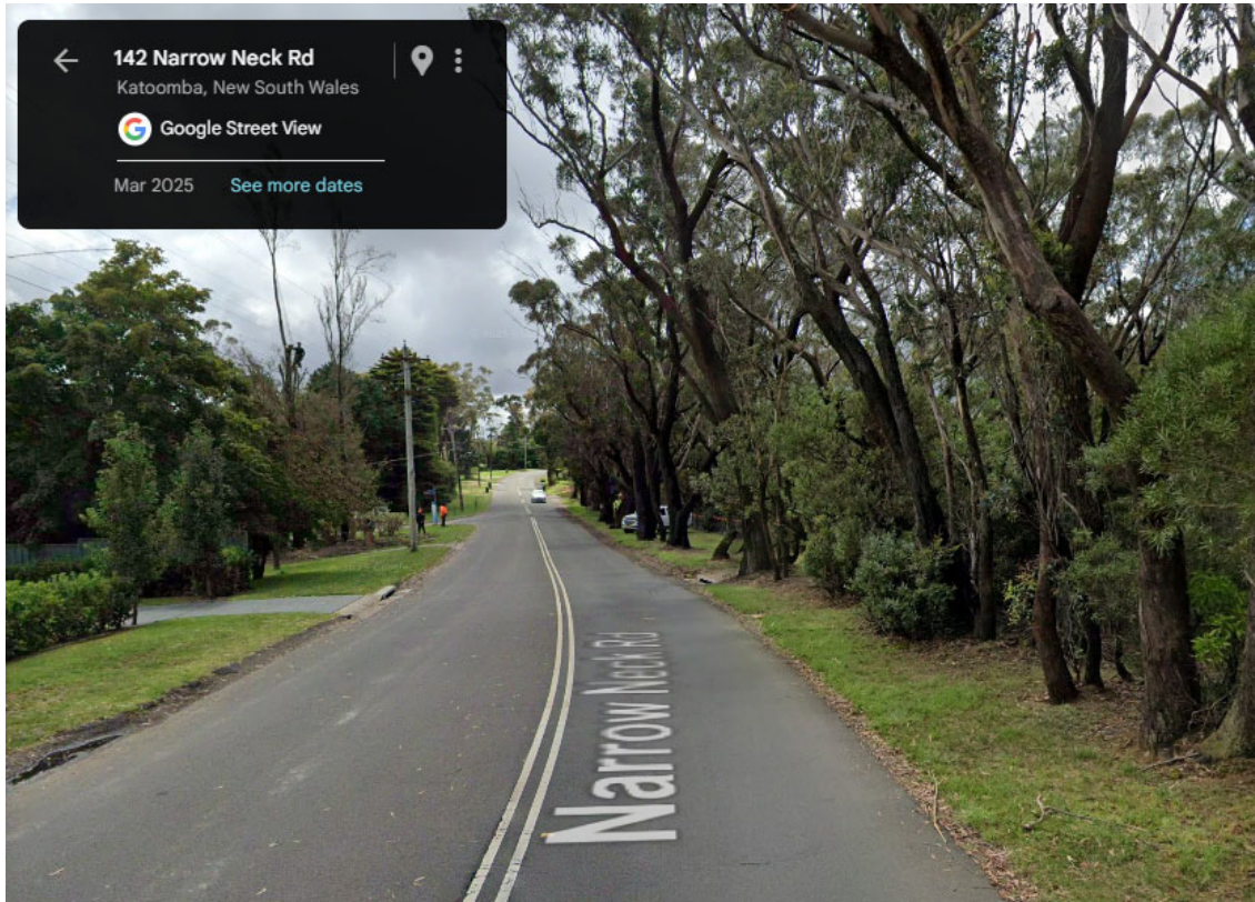
Figure 10: Evidence of road width and no footpaths adjacent to 142 Narrow Neck Road
