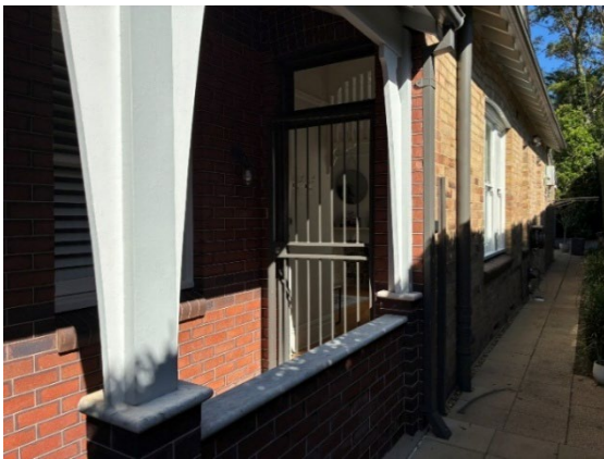
Side of 27 Rosalind Street (eastern boundary) – 22 March 3.30 pm
