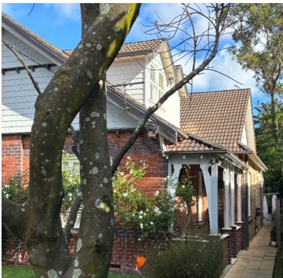
Side of 27 Rosalind Street (eastern boundary) – 23 March 4.30 pm
