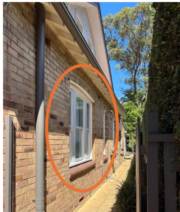
Side of 27 Rosalind Street (eastern boundary) – 22 March 1.30 pm
