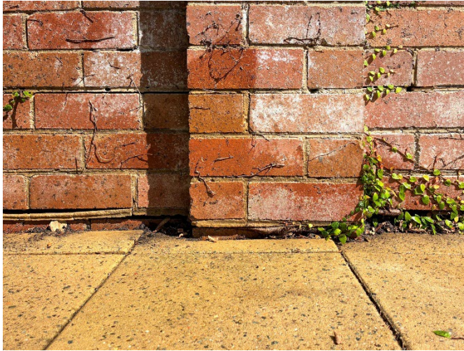
Brick sub-wall at the rear of 27 Rosalind Street (eastern boundary), supporting the developer's retaining wall:
