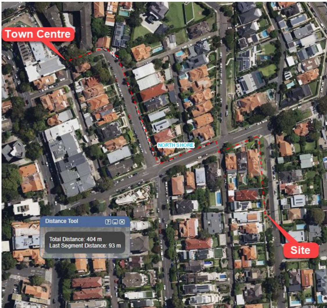
Figure 7 Correct Measurement of Green Line in Figure 13 of TIA relied upon by the EIS
