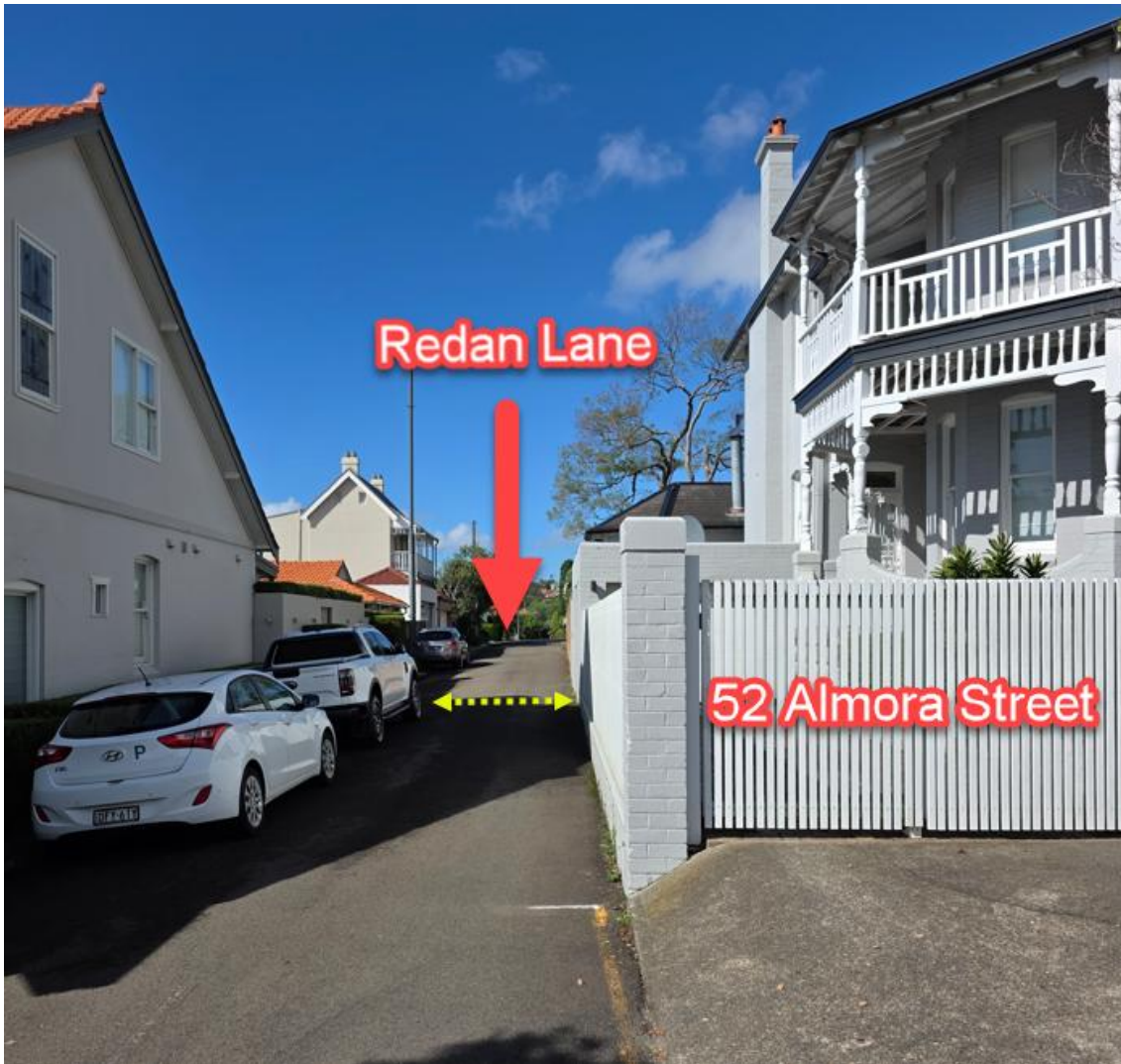
Figure 2 52 Almora Street (Heritage Item) and Narrow Redan Lane with No Pedestrian Footpath
