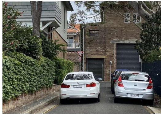
Photograph of Melaleuca Lane at the end of Muston Street. There is no path on the right and the kerb area on the left is not wide enough for pedestrians to walk along it. If a car comes, they need to turn sideways and step back.
