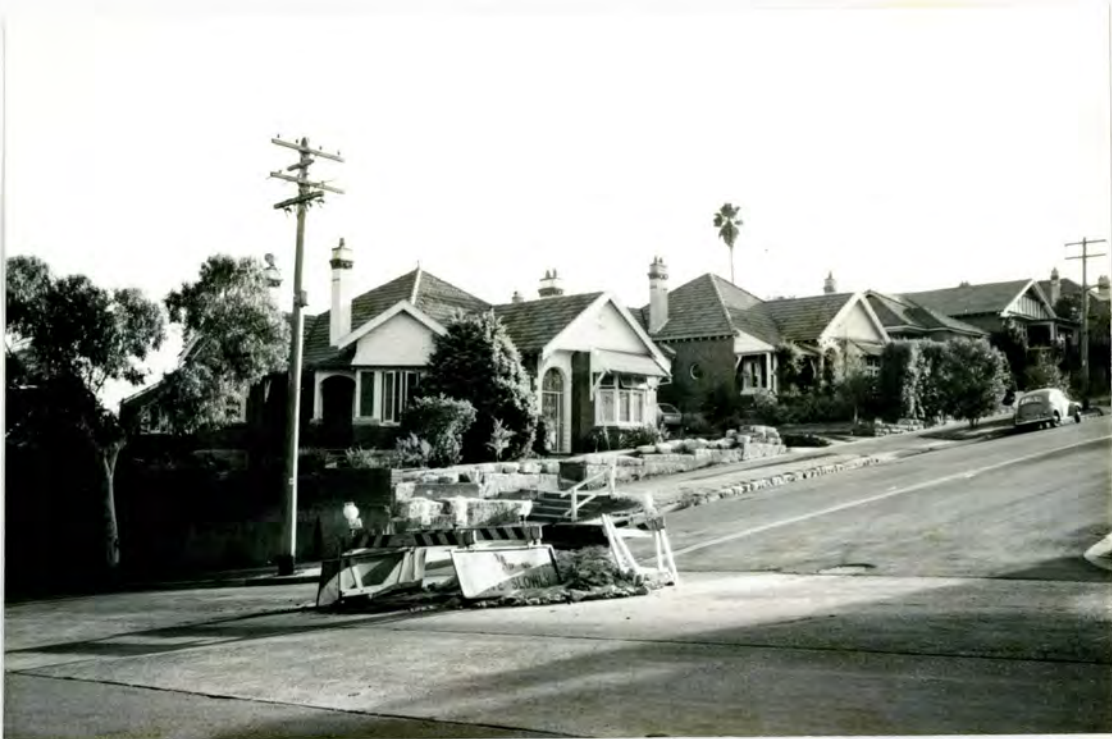
VIEW SOUTH - WEST FROM PARK ON SOUTH - EAST CORNER WOLGER AND COWLES ROADS TO INTERSECTION WITH SPENCER ROAD.
