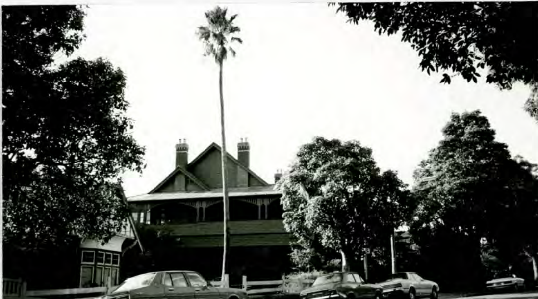
VIEW DUE NORTH TO NO. 20 BRADLEYS HEAD ROAD (WEST-SIDE OF ROAD)
