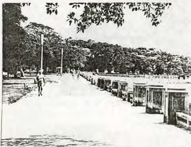
VIEW NORTH ALONG PROMENADE -NOTE WIDE WALKWAY AND TREE STREET
