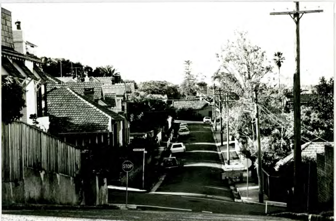
VIEW NORTH ALONG LITTLE STREET AND ACROSS MANDALONG ROAD TO LOWER PUNCH STREET.
