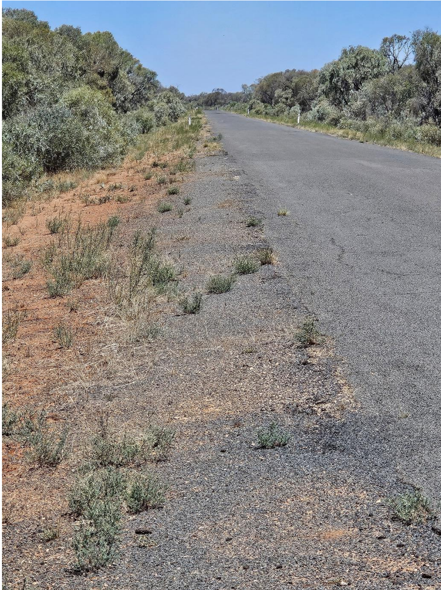
Figure 2 2km south of McLennons Bore Road and Cadell Road intersection looking south along Cadell Road
