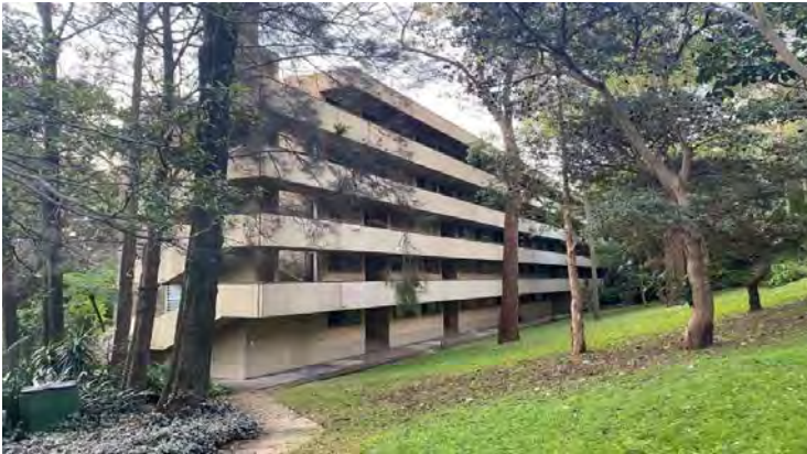
Figure 4.17: One of the site’s apartment complexes as viewed from the central lawn area, facing north. Source: Curio Projects 2022.
