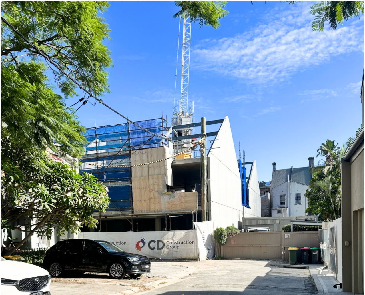
432–440 Oxford from rear. Currently under construction
