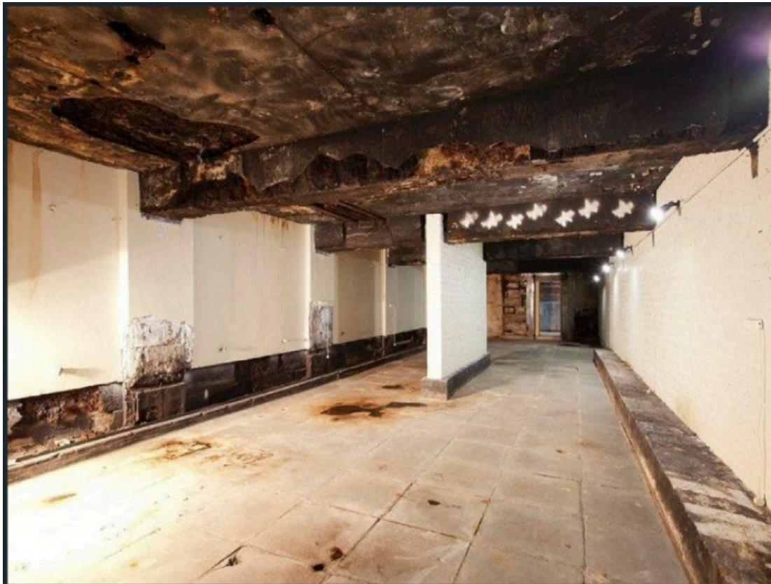
View of the historic Underground Basement below No. 142 Oxford Street Paddington, which predates the construction of the 1980s town house. Source: Photograph from the sale of No. 142 Oxford Street Paddington. Note the sandstone blocks under the render on the left hand wall. 2012. Source: realestate.com.au
