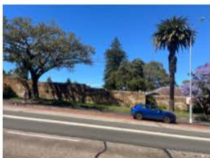
Fig. 98 The Victoria Barracks wall.
