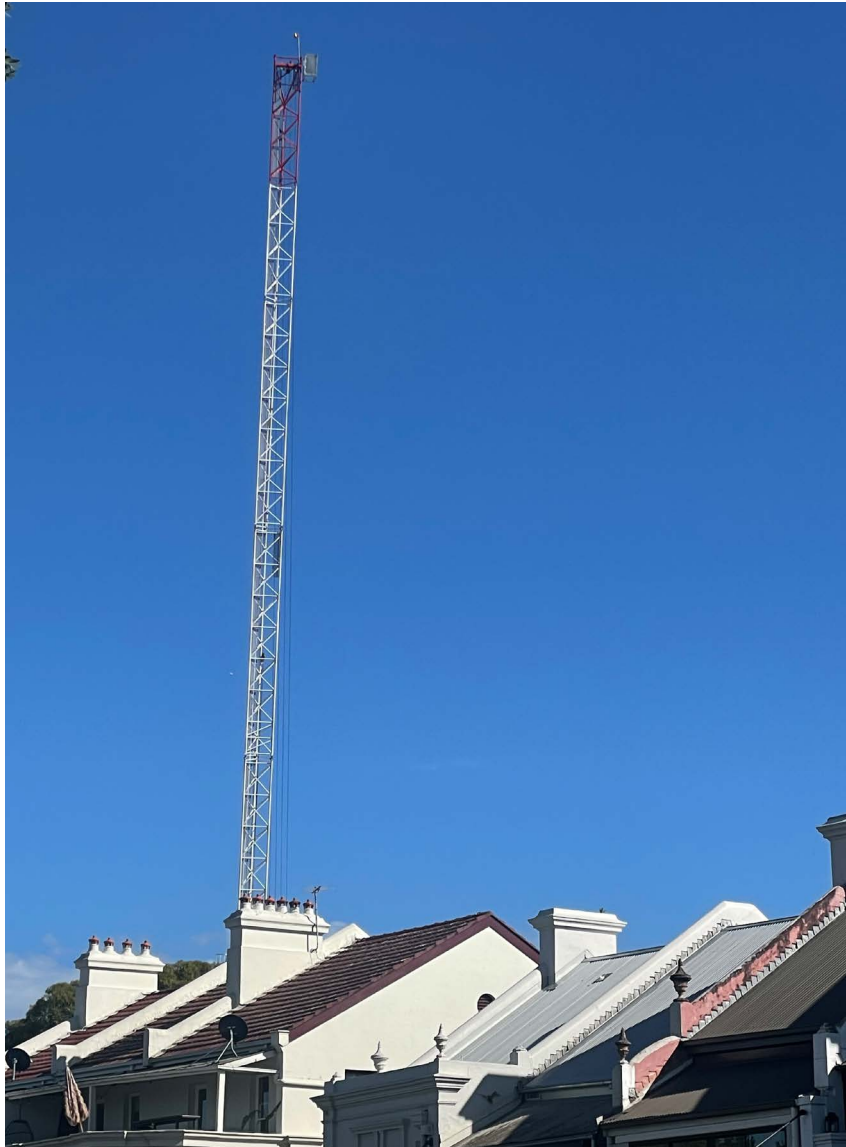
Oxford Street (Cambrian Construction)
