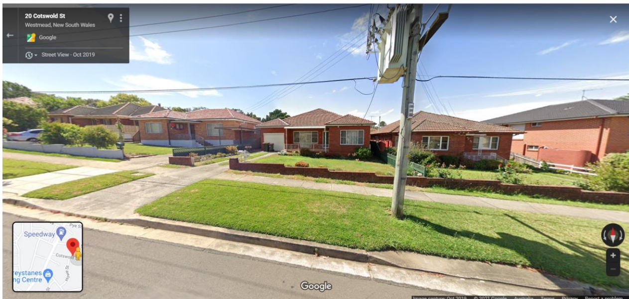
Driveways need to be appropriately located in relation to poles. Poles with transformers (pole mounted substations) may have an additional earth mat surrounding the pole and should be provided with greater separation to driveways. Repairs and maintenance to poles can occur over extended periods of time blocking driveway access. Source: Google Maps Street View.
