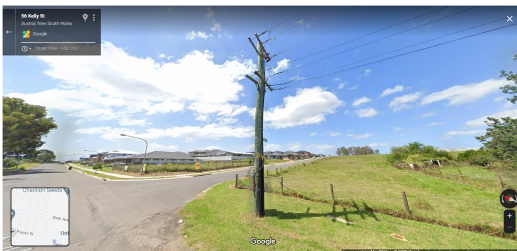
Overhead power lines are progressively undergrounded as subdivisions progress. Source: Google Maps Street View.
