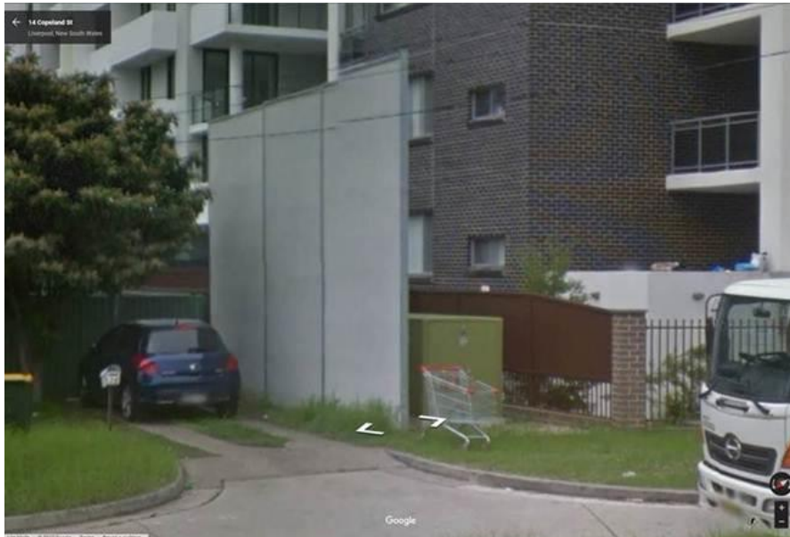
Fire wall constructed for padmount substation at 18 Copeland Street Liverpool. Source: Google Maps Street View.
