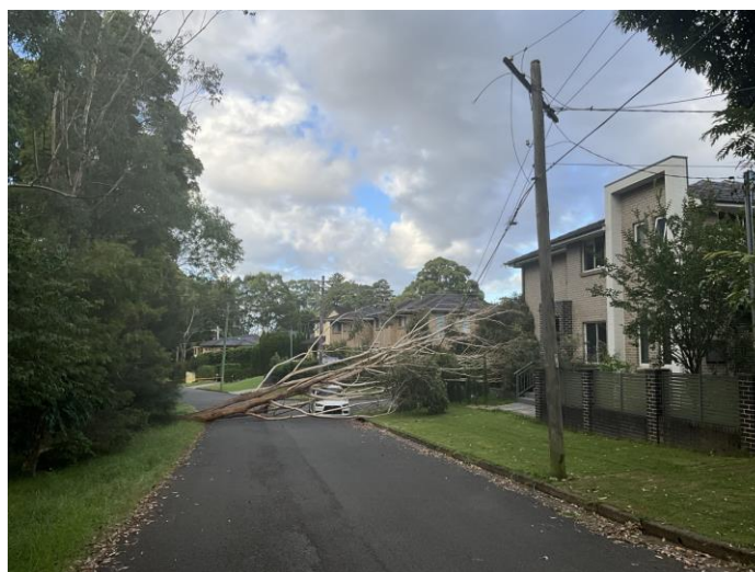
Although the spread of the tree on the opposite side of the road did not encroach safety clearances to the overhead power lines, the height meant that when the tree fell during a storm, it damaged the overhead power lines requiring repairs to restore electricity supply to customers. Source: https://web.yammer.com/main/org/endeavourenergy.com.au
