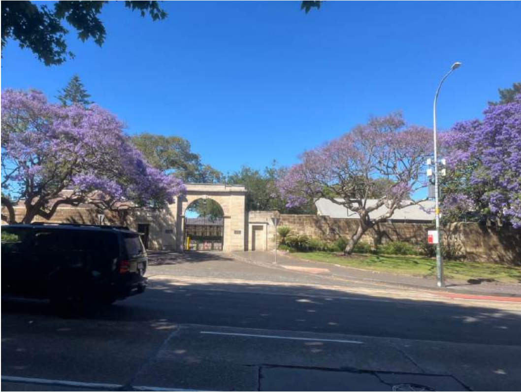
Fig.56 Victoria Barracks Wall and gate
