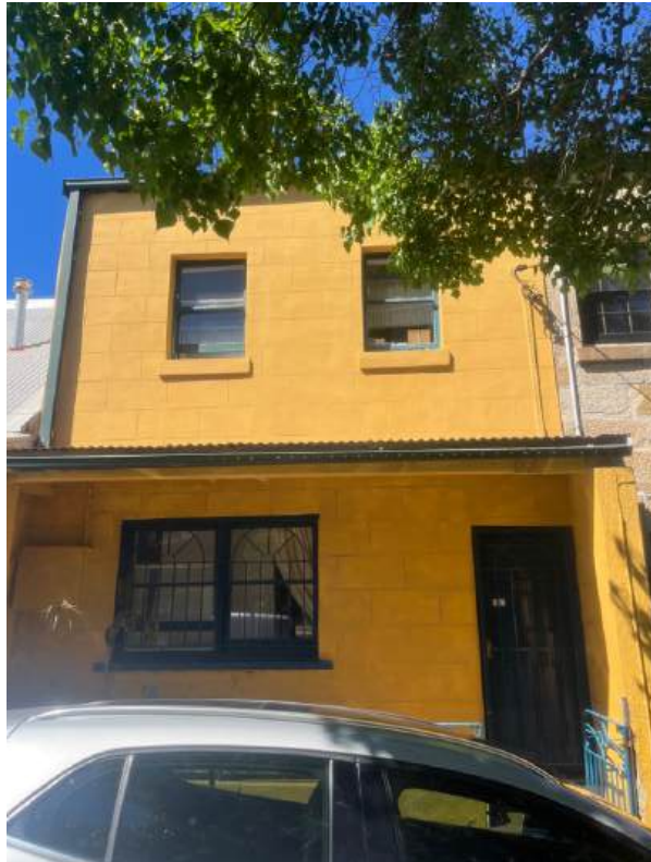
Fig.85 Mid-Victorian terrace Gipps Street
