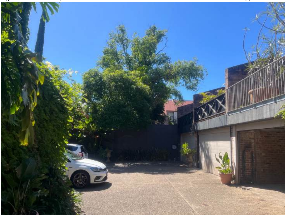
Fig.80 Access to carparks at 142-148 Oxford Street is from a narrow Lane from Gipps Street.
