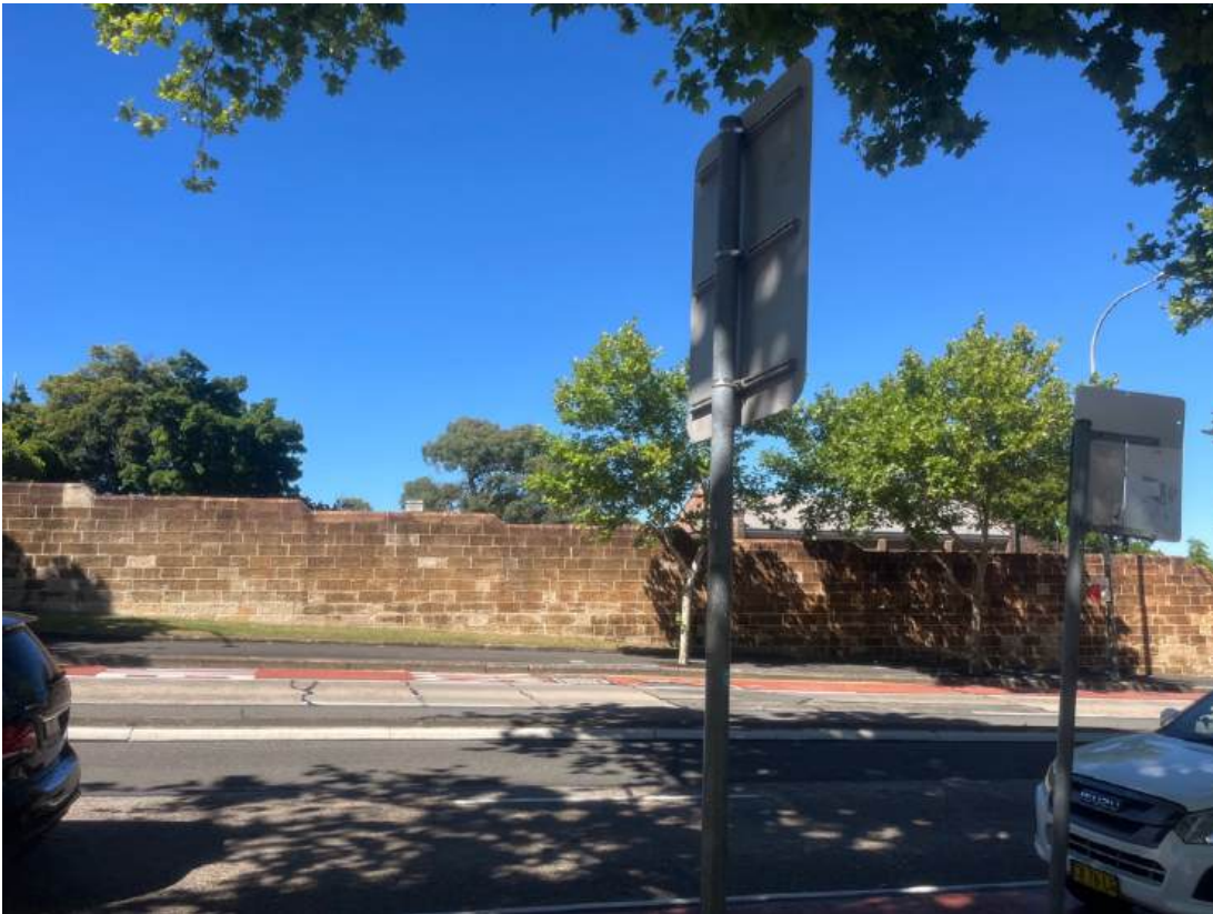
Fig.46 Victoria Barracks wall
