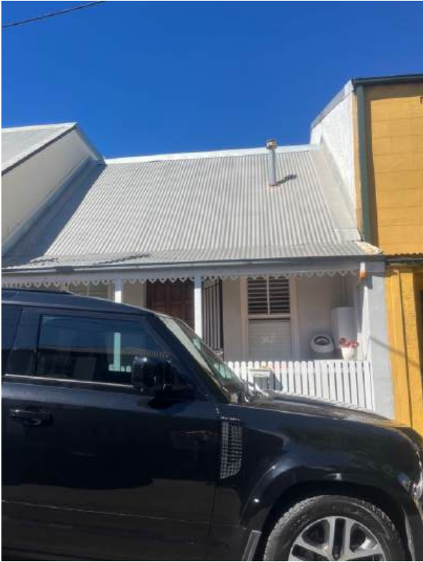
Fig.86 Cottage on Gipps Street
