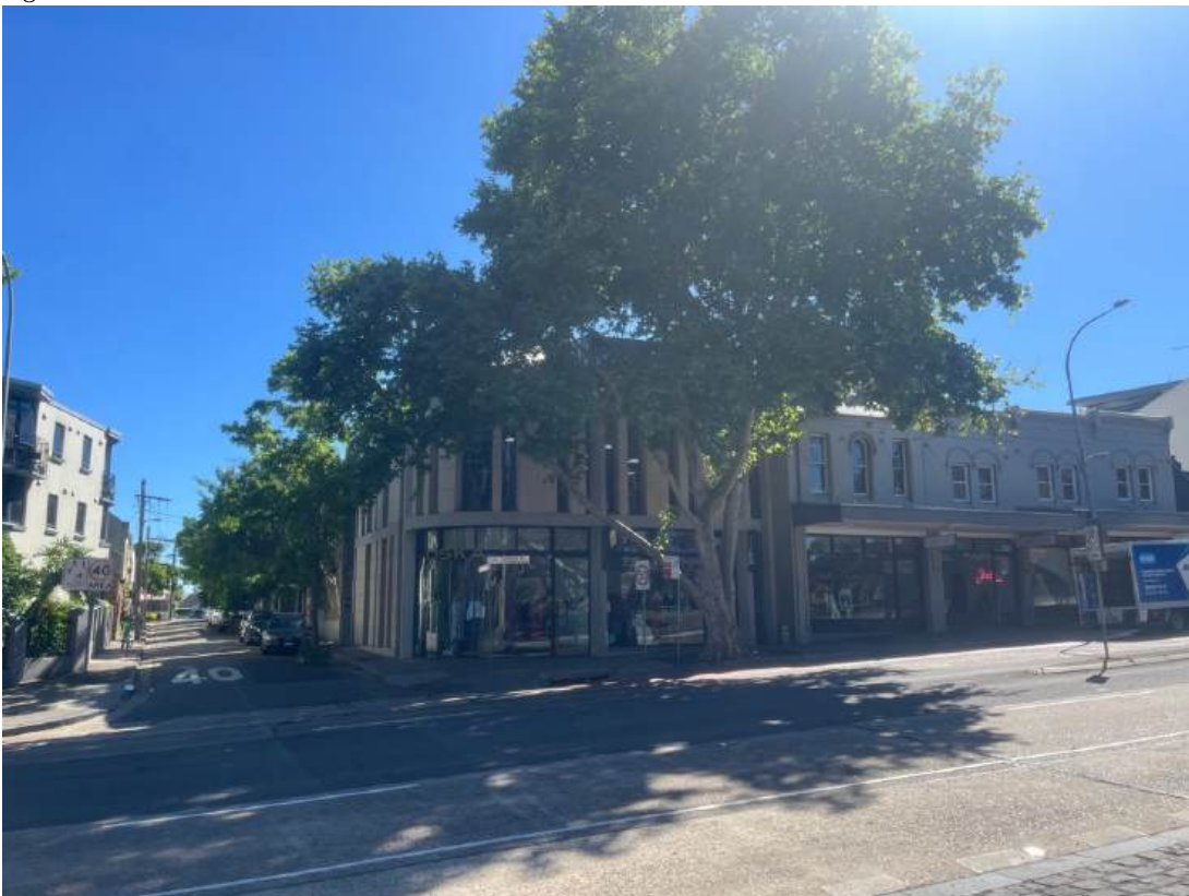
Fig.11 No. 162 Oxford Stree contains a shop with offices above. It is beside a Federation commercial terrace.
