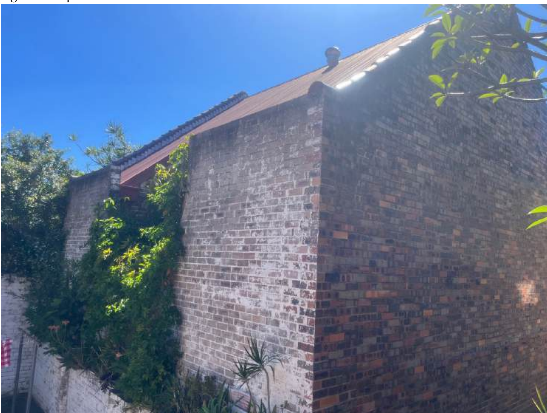
Fig.106 Rear wall of No. 6 Shadforth Street from rear of No 160 Oxford Street.
