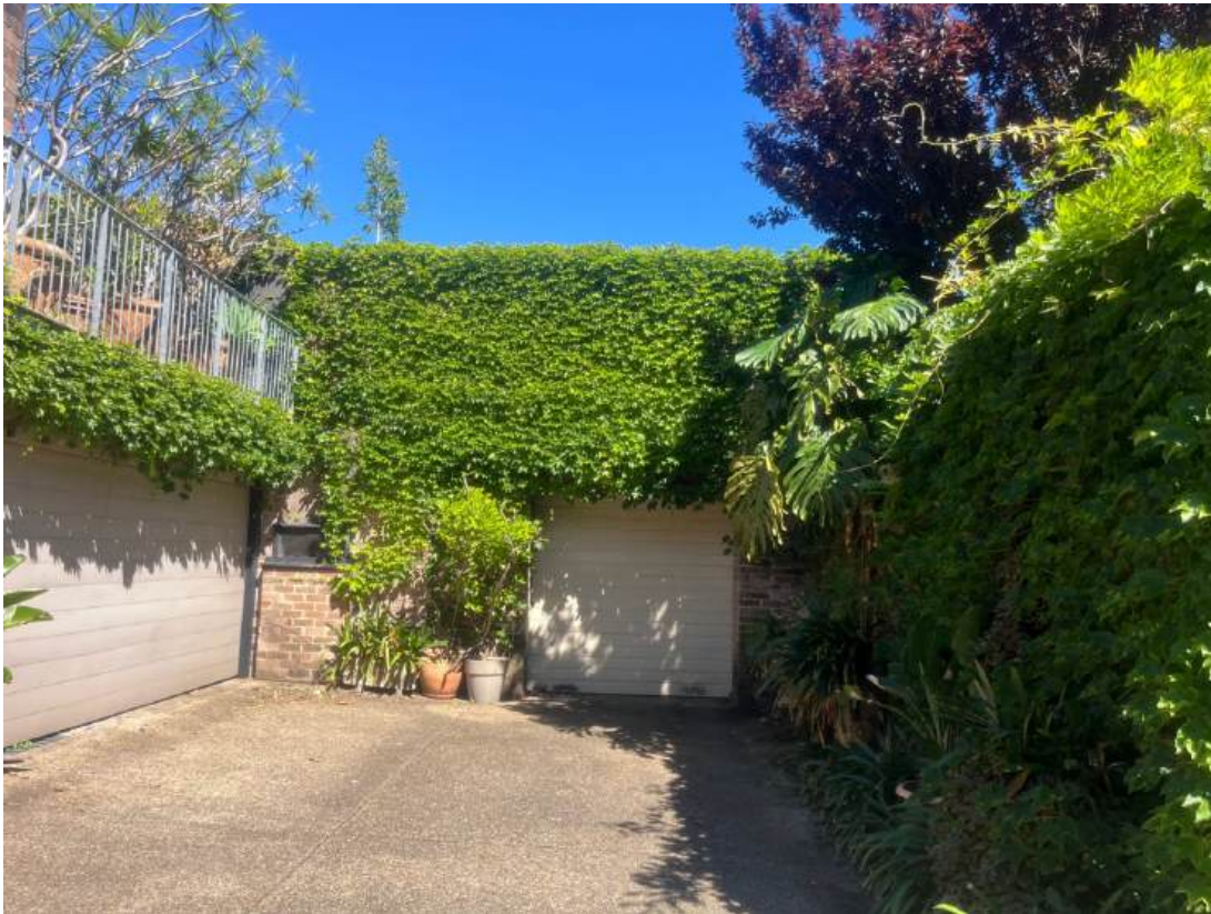
Fig.77 Carpark access at rear of Nos.142-148 Oxford Street.
