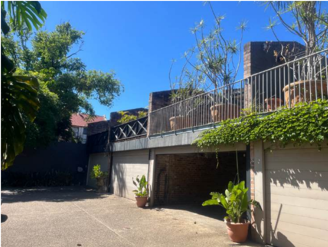
Fig.79 Access to carparks at 142-148 Oxford Street is from a narrow Lane from Gipps Street.
