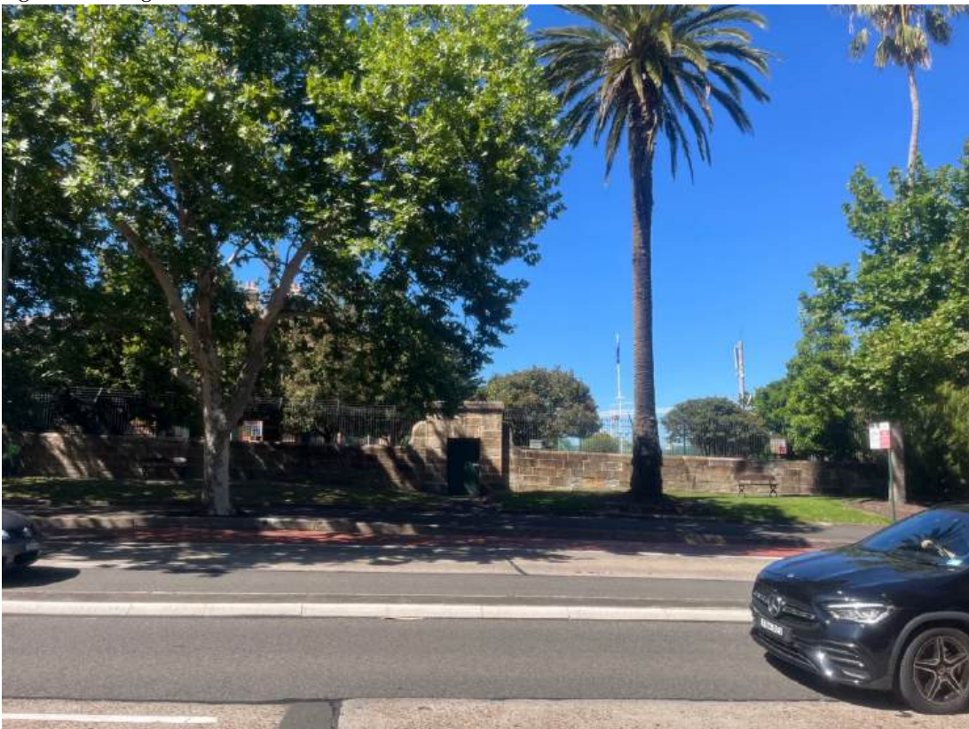
Fig.43 Victoria Barracks wall
