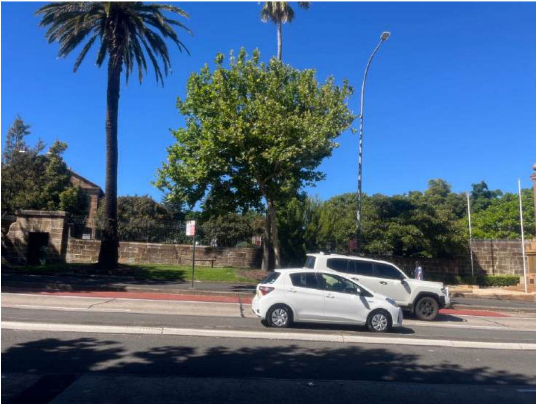
Fig.44 Victoria Barracks wall
