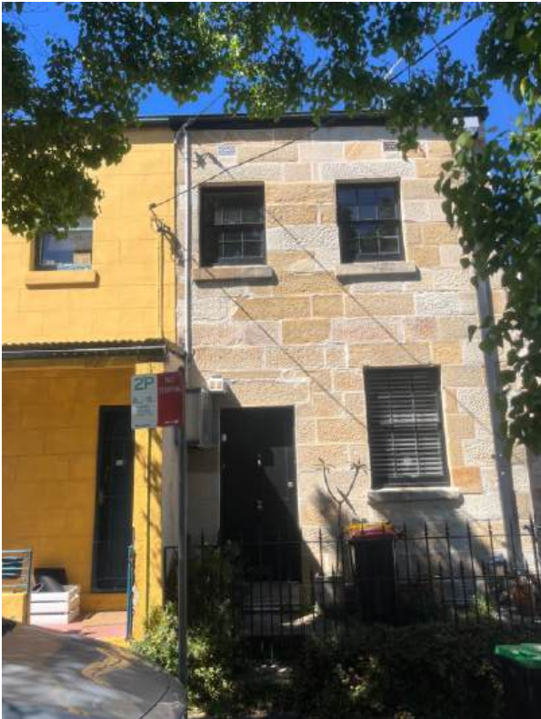
Fig.84 Mid-Victorian terrace Gipps Street
