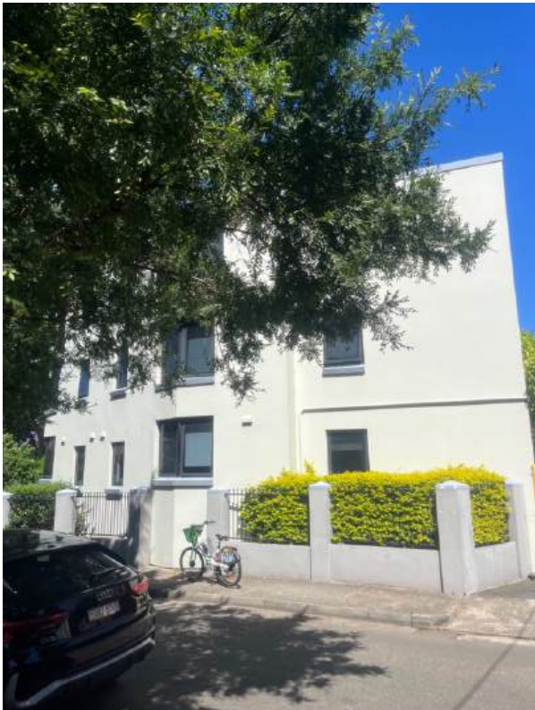
Fig.93 Shadforth St façade of 160 Oxford St
