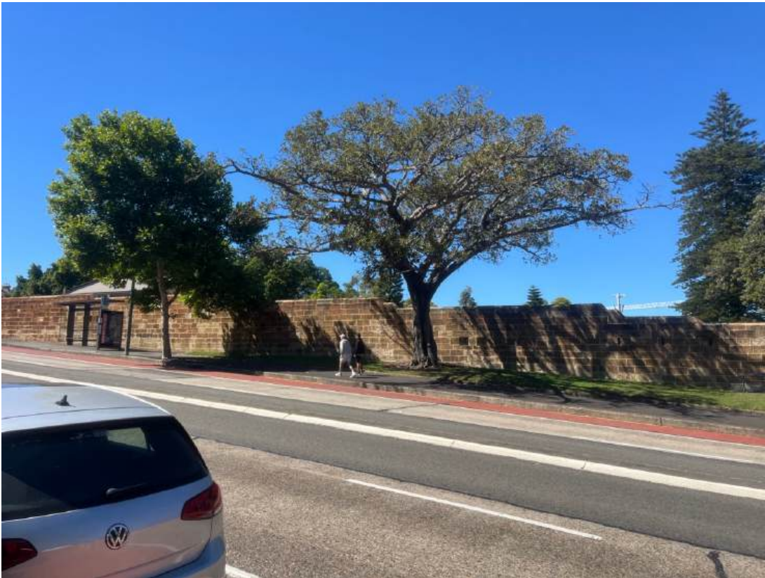
Fig.52 Victoria Barracks Wall
