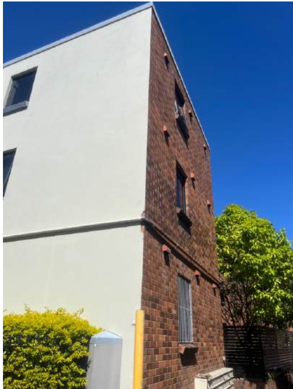
Fig.94 Shadforth St and rear façade No. 160 Oxford Street
