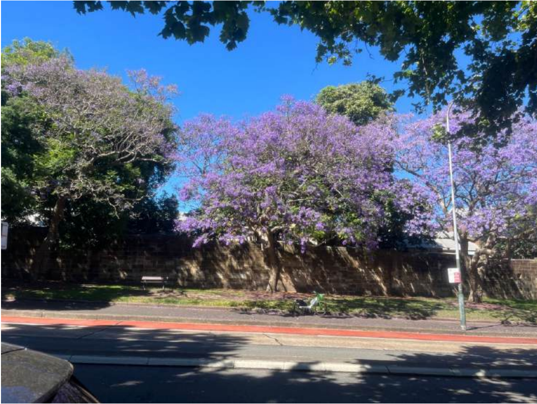
Fig.60 Victoria Barracks Wall
