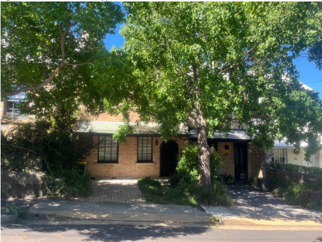
Fig.70 19, 17, and 15 Gipps Street are terraces built in the 1870s
