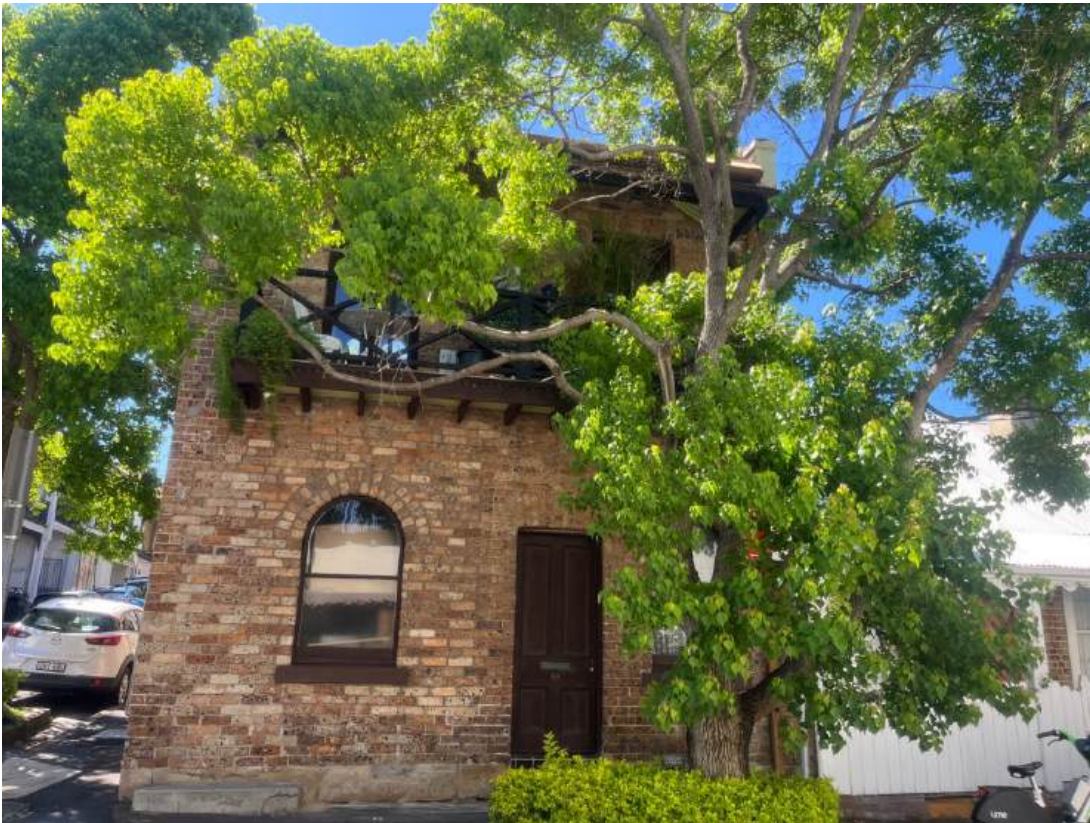
Fig.115 This house on the east side of Shadforth Street was a corner shop. A sign for Zyp lemonadae is prominent in Gipps street
