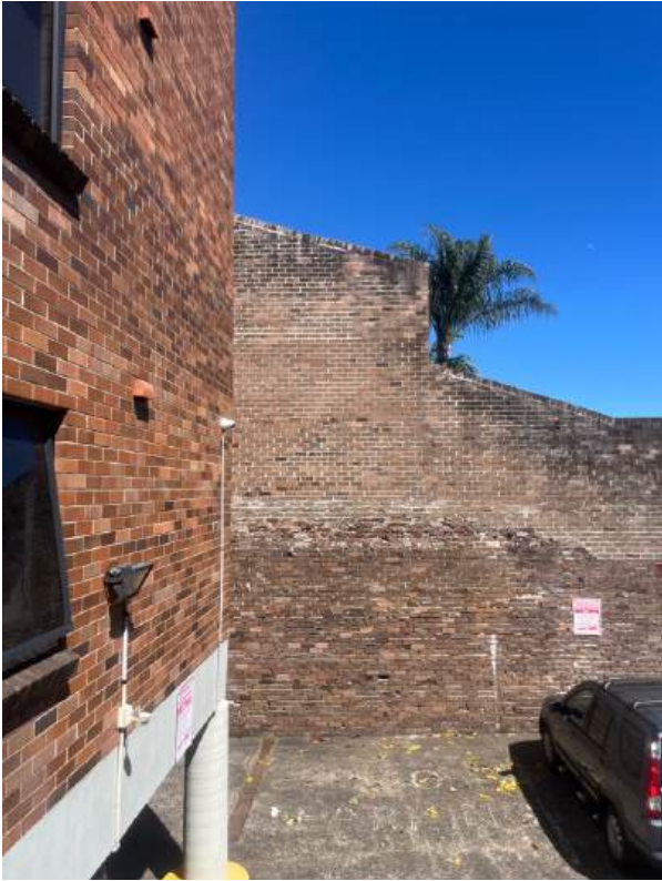
Fig.103 Carpark for units at 160 Oxford Street
