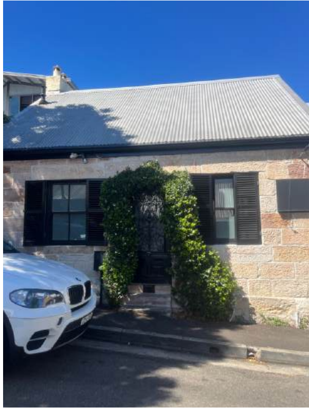
Fig.87 Cottage on Gipps Street
