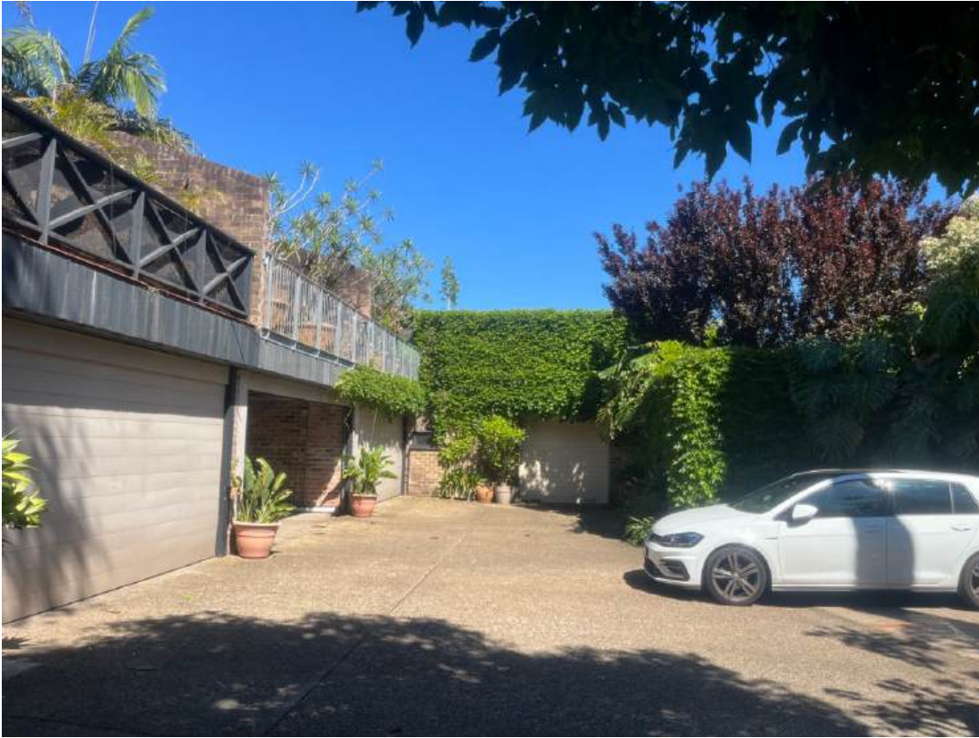
Fig.81 Access to carparks at 142-148 Oxford Street is from a narrow Lane from Gipps Street.
