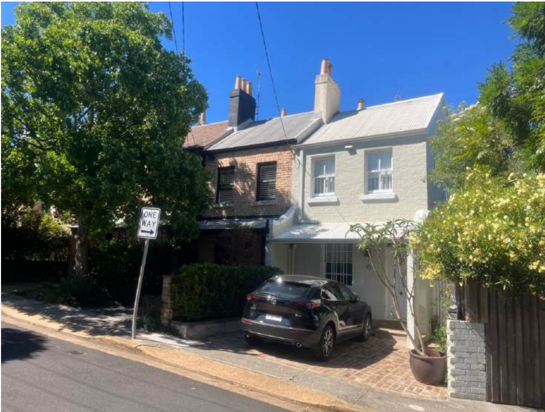
Fig.69 Nos. 19, 17, and 15 Gipps Street is a terrace built in the 1870s
