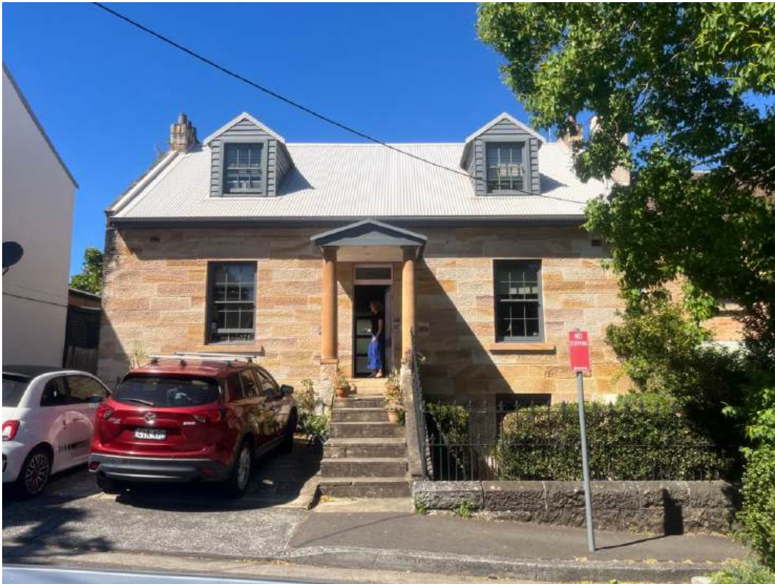
Fig.71 The original Paddington Police station No 21 Gipps Street
