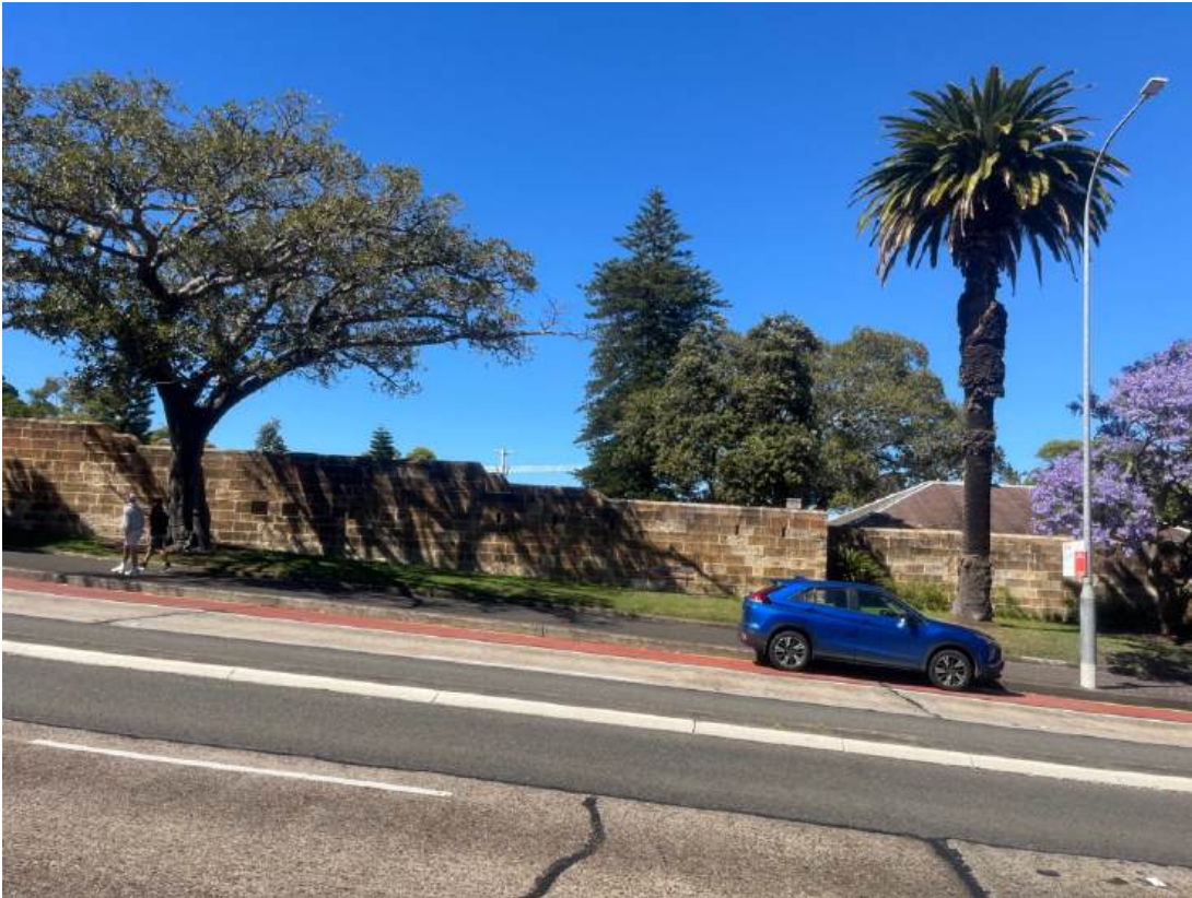
Fig.51 Victoria Barracks Wall
