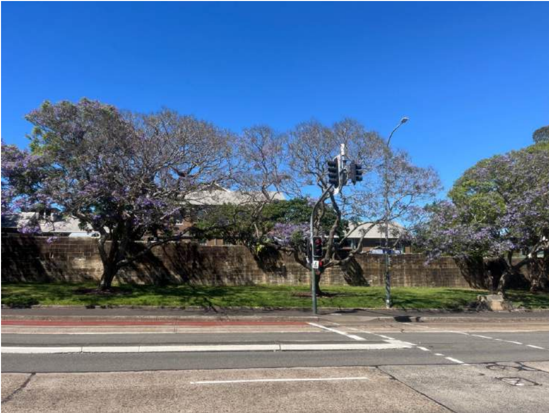
Fig.61 Victoria Barracks Wall
