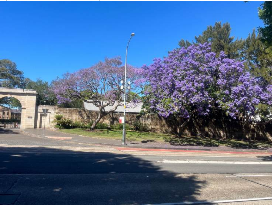
Fig.57 Victoria Barracks Wall and Gate
