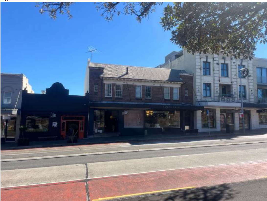
Fig.13 Row contains a baker and delicatessen, a Federation building and the Greenwood Tree Hotel. Now units.
