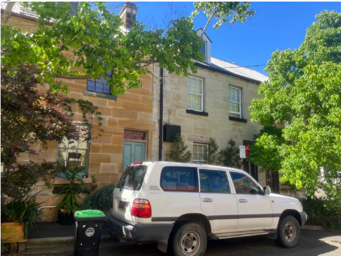
Fig.112 These larger sandstone houses on Shadforth Street denote a higher rank of the occupants. Skilled tradesmen or foremen.
