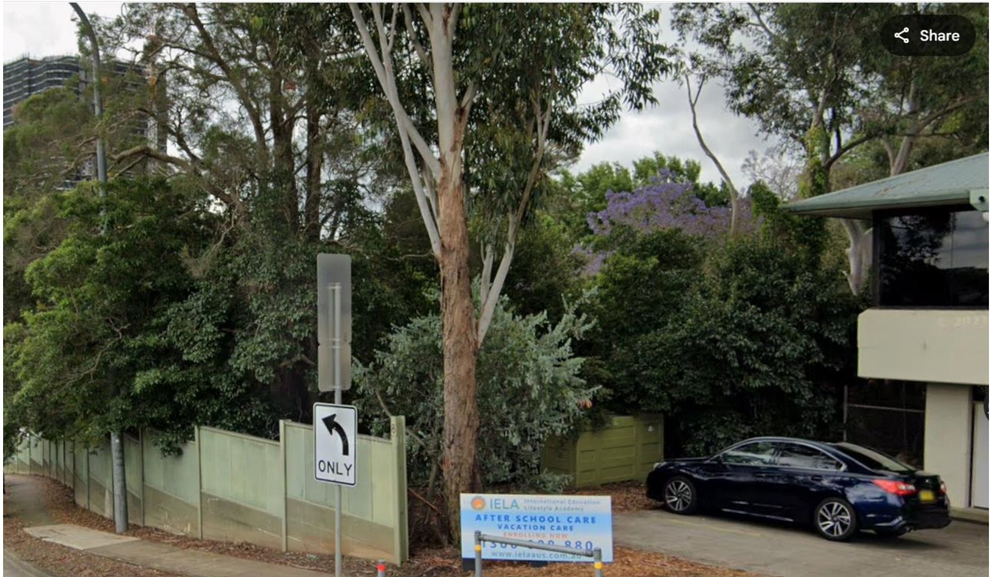
Google Maps Street View. Padmount substation no. 17198.
