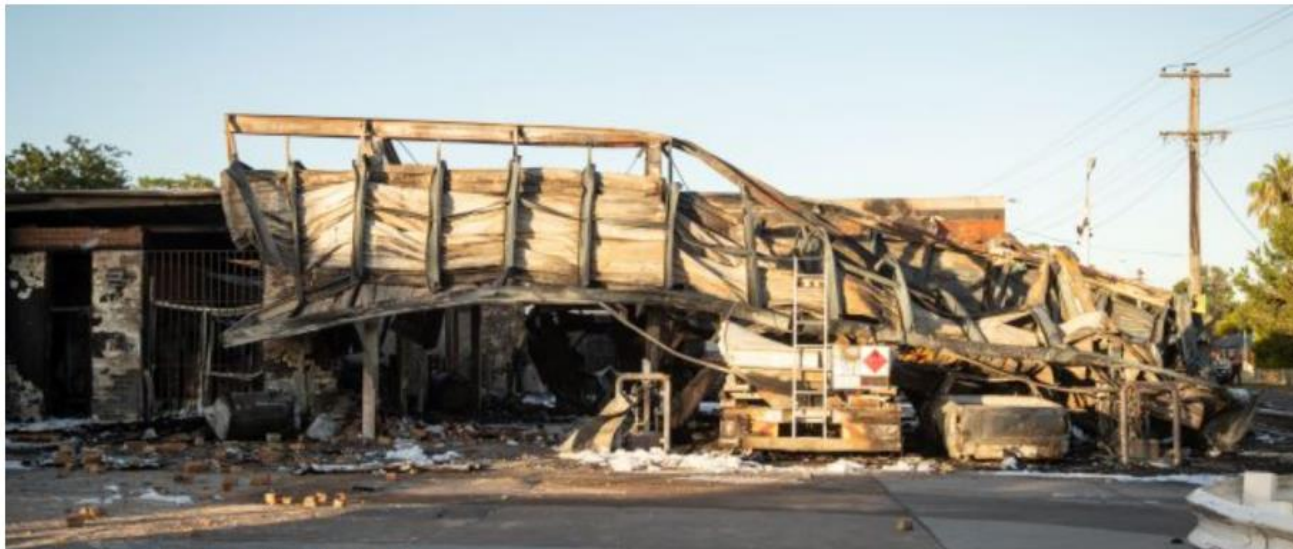
Figure 4: Service Station Facility Following Fire
