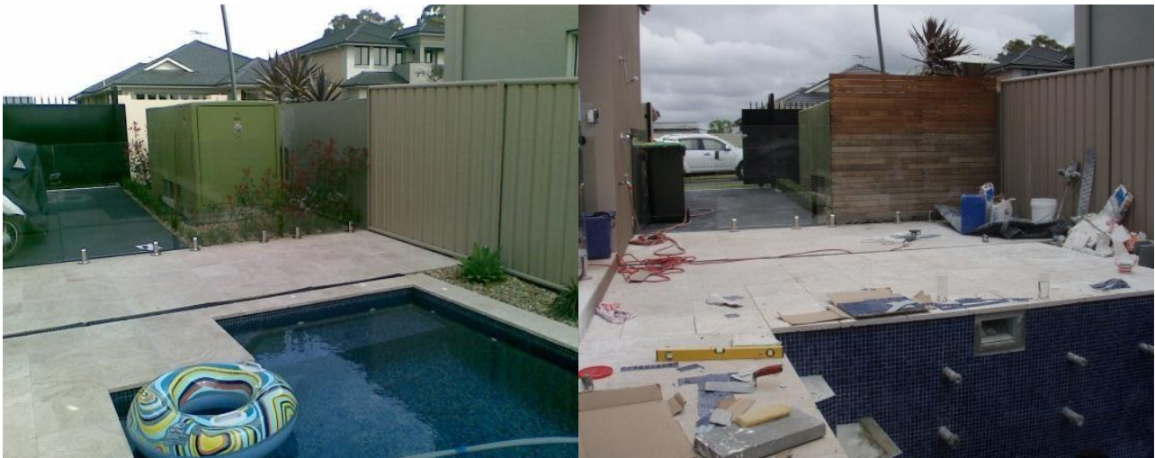
Before and After. This swimming pool in Endeavour Energy's network area at Middleton Grange NSW had to be modified to comply with the restriction for the padmount substation on the use of land in relation to swimming pools.
