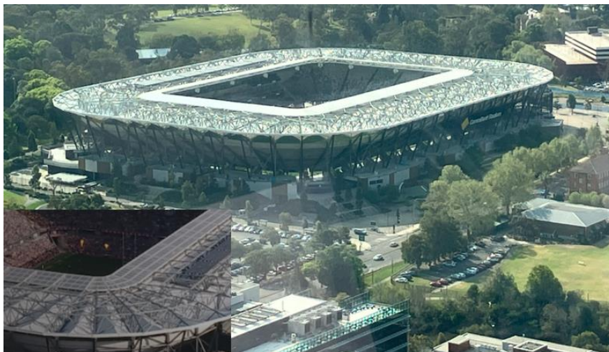
The roof at Bankwest (now CommBank) stadium in Parramatta supports a 100 kilowatt hour (kWh) solar panel system 309 individual solar panels generating renewable energy for the stadium. Source: Bankwest Stadium Sustainability Case Study May 2020.
