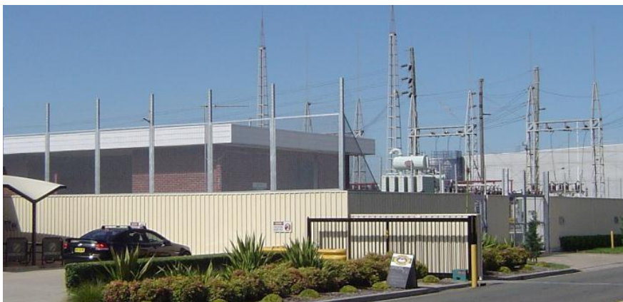
Endeavour Energy's Seven Hills Zone Substation is an 'outdoor' design. Note height of fencing due to adjacent 'climb point' created by the seating and awning. Source: Google Maps Street View.
