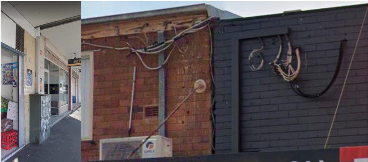
Example of 'awning' overhead power lines coming from a low voltage pillar on the road verge rising to through a duct and then through or above the awnings to the customer connection points for the premises. Source: Google Maps Street View.
