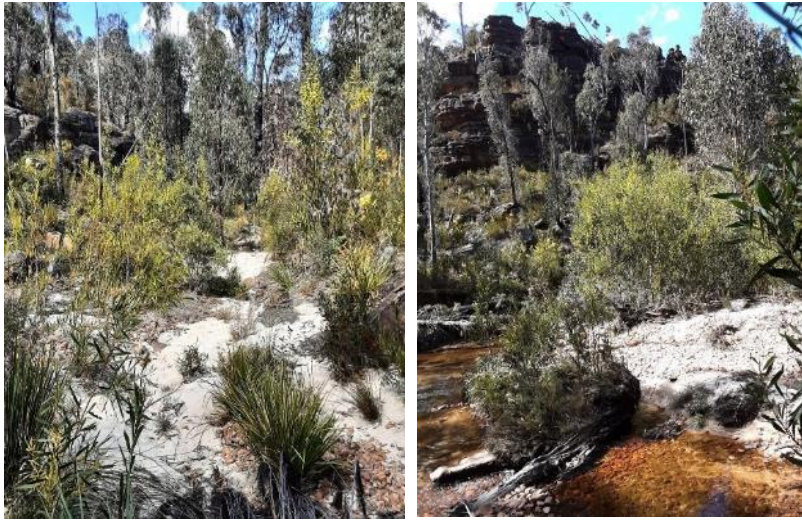
Photo 50 & 51: Bungleboori Creek tilted by Panel 606 & forming a new channel
