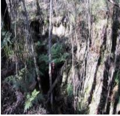
Photo 4: Site 1 Sinkhole – July 2010
