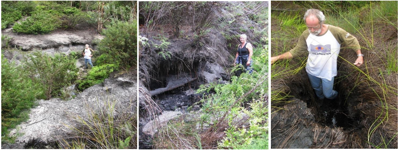
Photos 36, 37, 38: Site 12 – Erosion, channelization, slumping downstream of Clarence Transfer discharge – 31 January 2010
