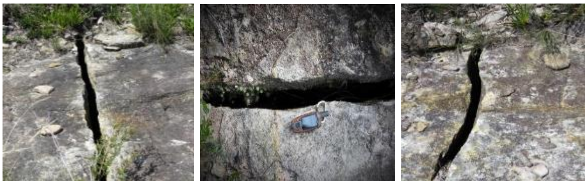
Photo 1, 2, 3: Mine subsidence cracks on Kamarah Ridge and Jungaburra Ridge above Canyon Colliery – 10 February 2015
