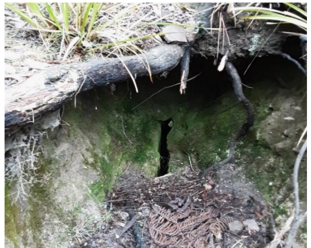
Photo 2: Site 1 Subsidence crack in sinkhole - June 2024
