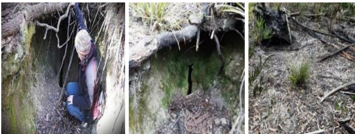
Photo1: Site 1 Crack in sinkhole - July 2010 Photo2: Site 1 Crack in sinkhole June 2024 Photo 3: Dry creek downstream 2024
