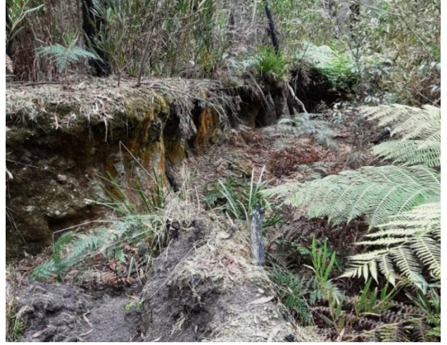
Photo 4: Site 1 Mine subsidence sinkhole – June 2024
