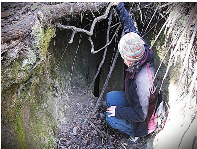
Photo 1: Site 1 Subsidence crack in sinkhole - July 2010
