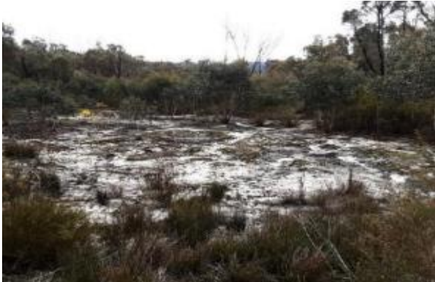
Photo 7: Site 2 Damaged THPSS – June 2024
