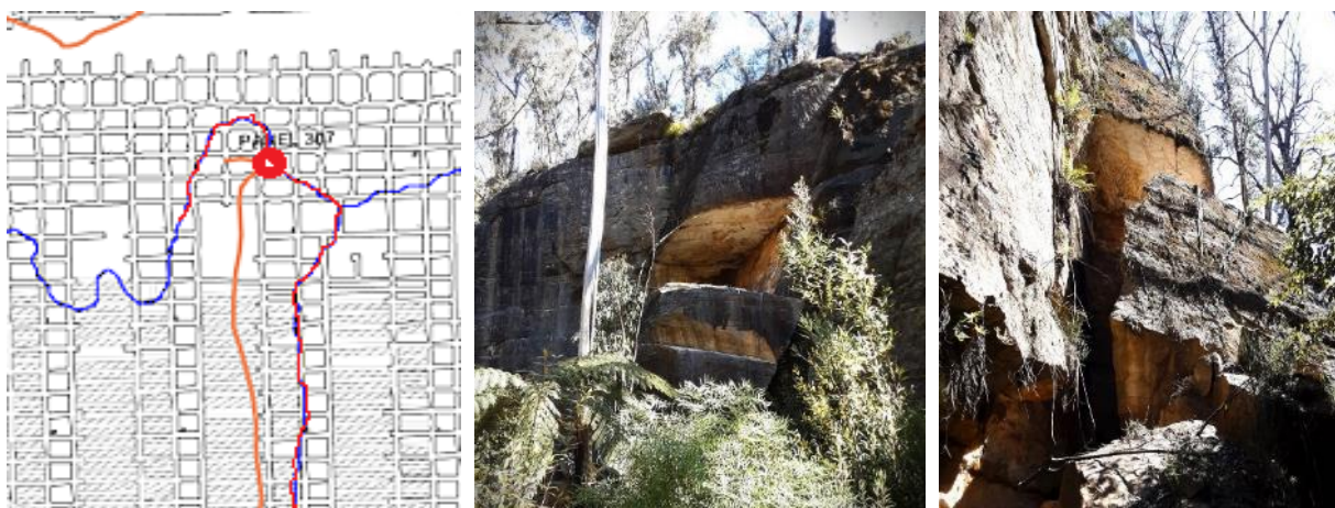
Figure 4: Rock fall (red dot), dry creek
