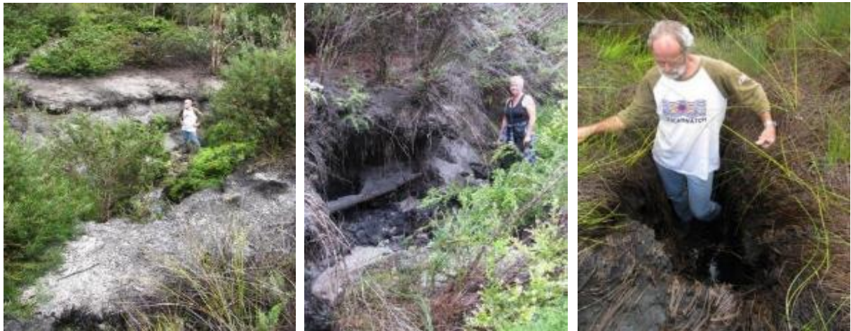
Photos 37, 38, 39: Site 12 – Erosion, channelization, slumping downstream of Clarence Transfer discharge – 31 January 2010
