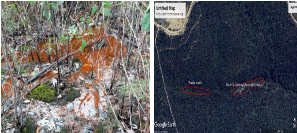
Photo 32 & 33: Site 1 1- Rusty-red discoloured water & swamp damage Longwall 1 – June 2024
