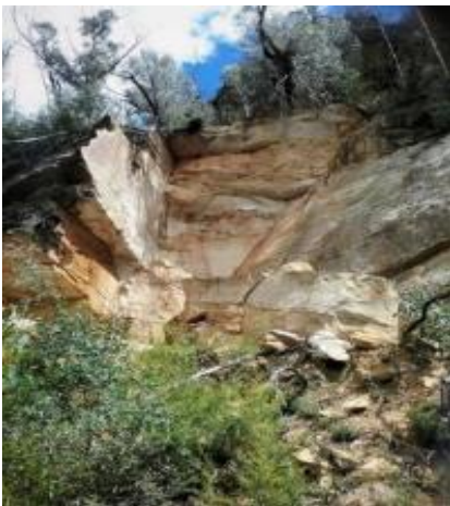
Photo 29: Cliff collapse - Panel 912
