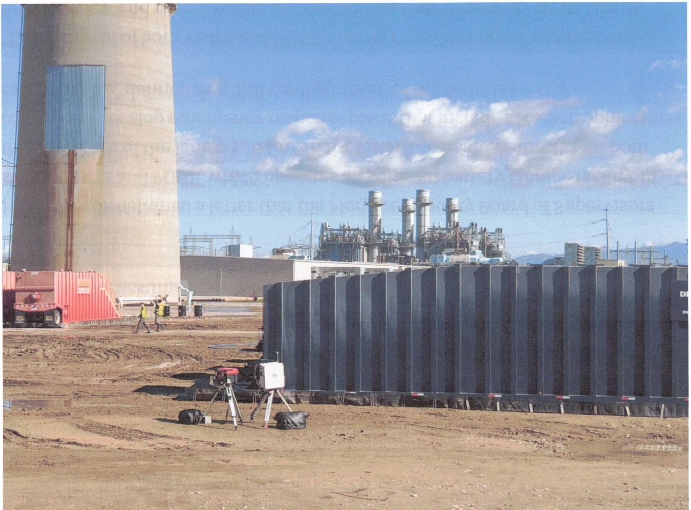
Cleanup crews and vehicles are in place at the Vistra Moss Landing battery storage facility on February 8, 2025, at Moss Landing, Calif. Source: Ruth Dusseault/Bay City News
