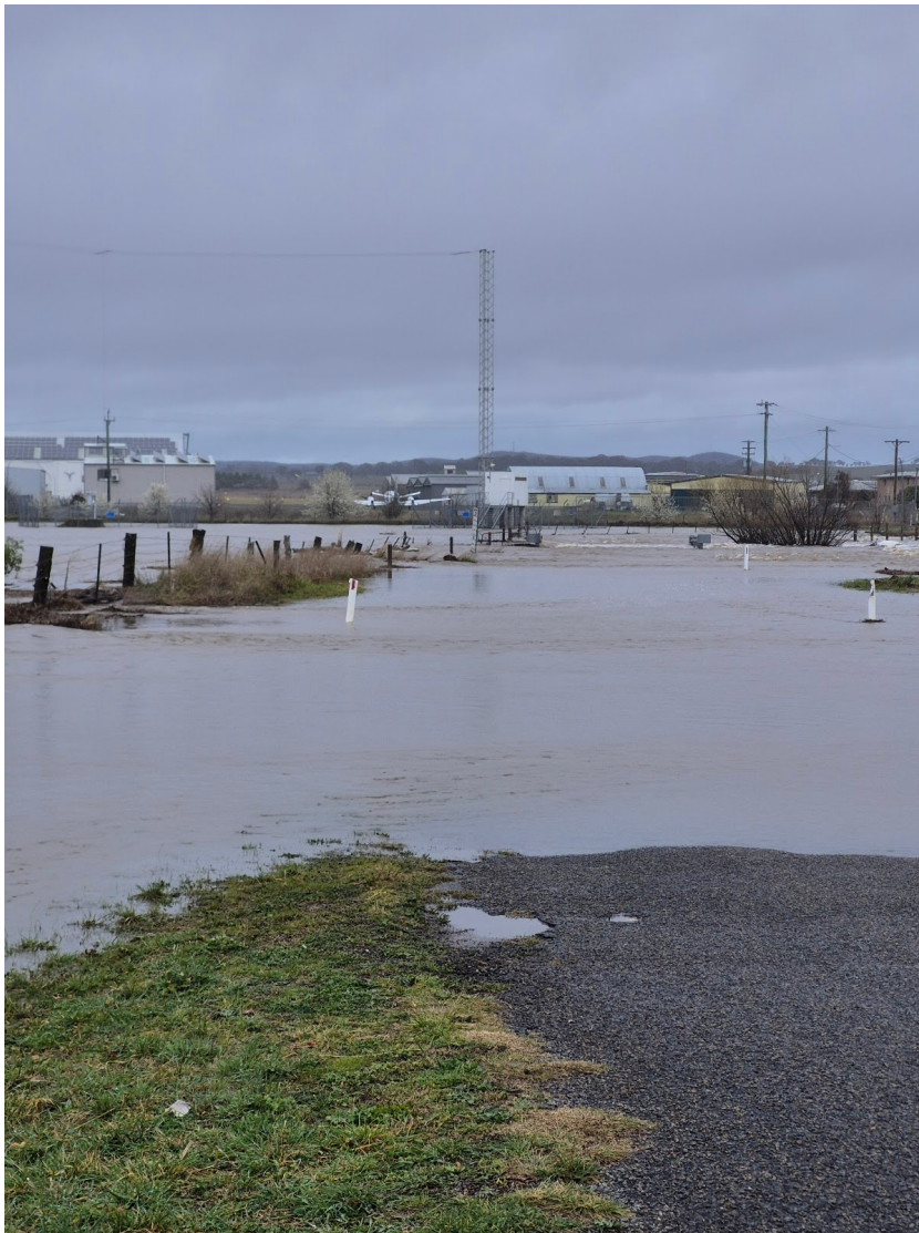
Airport Lane Closed due to flooding. Cumulative effect from both Merino & Gundry Solar Farm catchment areas
