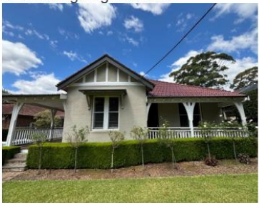
27 Roseville Avenue, Primary façade with extensive alterations
