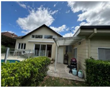
25 Roseville Avenue, Contemporary rear extension
