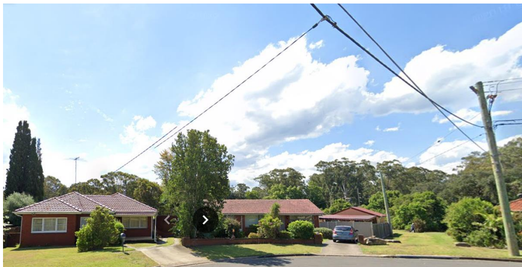
Mid span / suspended low voltage overhead service conductor for a dwelling at Rydalmere. Source: Google Maps Street View.
