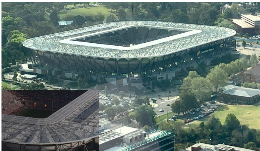
The roof at Bankwest (now CommBank) stadium in Parramatta supports a 100 kilowatt hour (kWh) solar panel system 309 individual solar panels generating renewable energy for the stadium. Source: Bankwest Stadium Sustainability Case Study May 2020.
