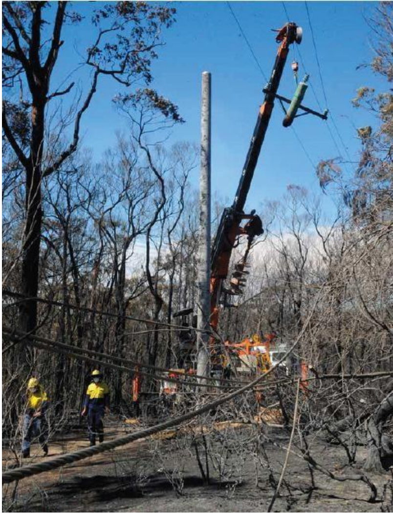
Endeavour Energy crews replacing a burnt timber pole with a concrete pole after the September 2013 bush fire at Winmalee NSW. Source: Everyday Endeavours, Staff Newspaper November 2013
