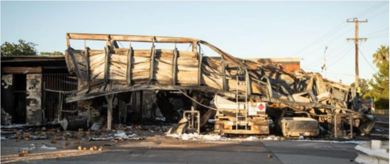
Figure 4: Service Station Facility Following Fire
