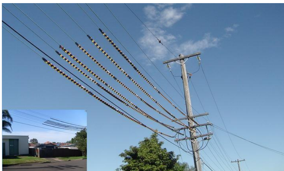
'Tiger Tails' are used primarily as a visual indicator or for mechanical protection from electrical wires. They are not to be used as insulating material and will not provide full protection from live electricity. This example is of tiger tails installed by Endeavour Energy on overhead power lines at Ermington NSW as part of a risk management for work on a nearby Distribution Substation No. 20981. Source: Google Maps Street View.
