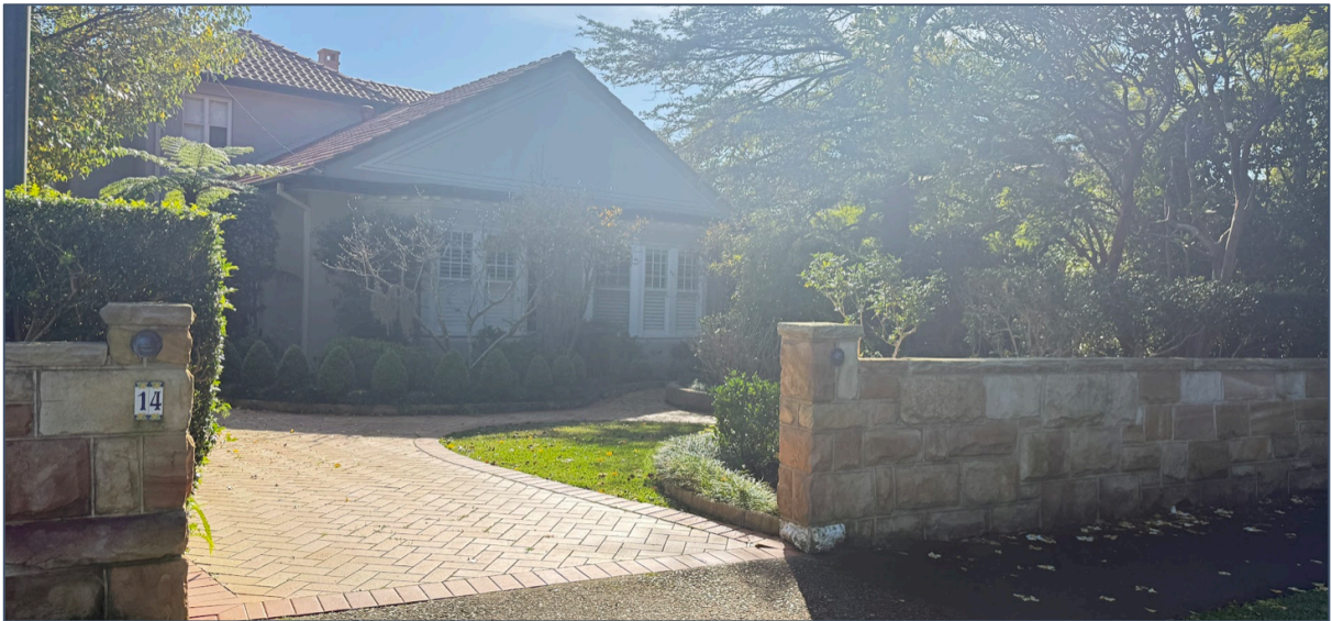
Figure 3 – Development site viewed from street (Corona Projects, 2025)
