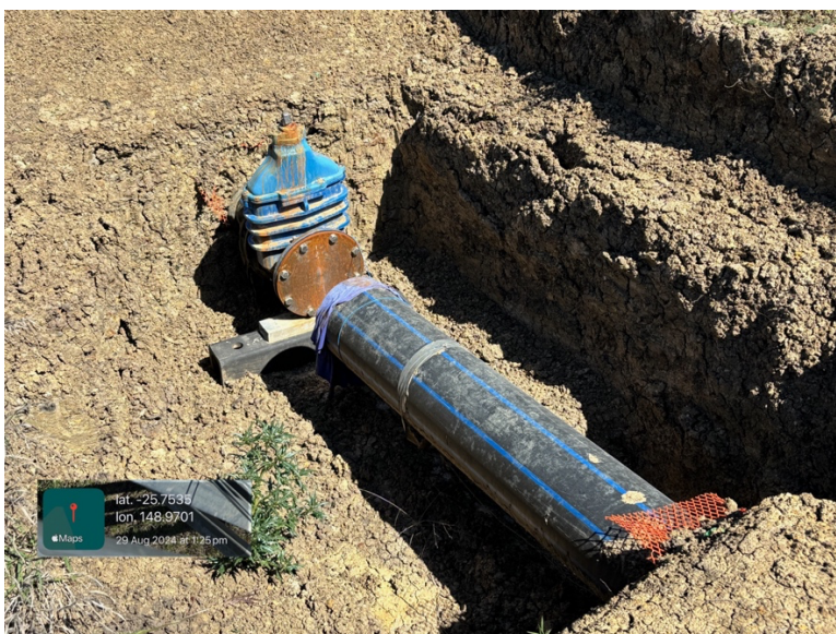
A gathering line is exposed to be repaired, Hallett State Forest, QLD
