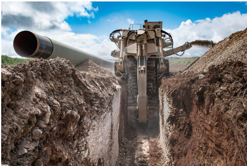
A typical pipeline trencher
