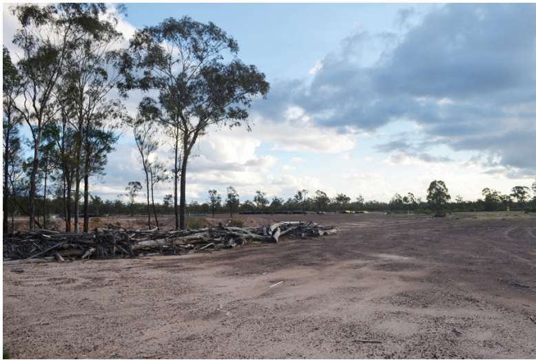
A laydown yard in south-west Qld
