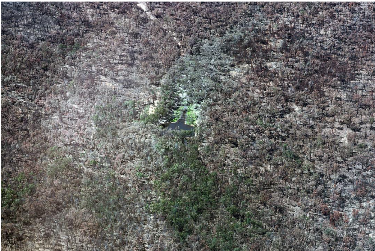
Yellow Spring Dam shortly after the Duck Creek Fire. Image courtesy of Wando CCC
