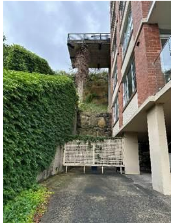
Image illustrating buildings at the base of the cliff edge on Park Avenue, some constructed on pylons that would be vulnerable to strong vibrations caused by bulk excavation works (taken on 12/12/2025).
