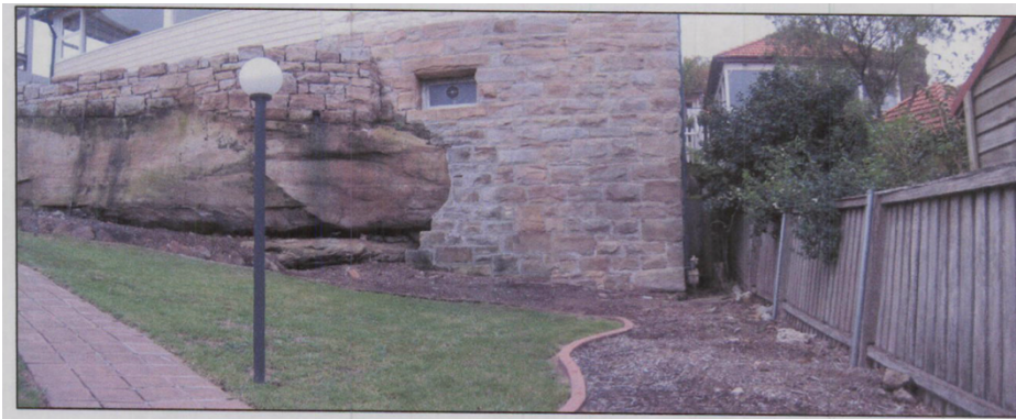
Photo 4 Existing foundation wall and rock cutting
