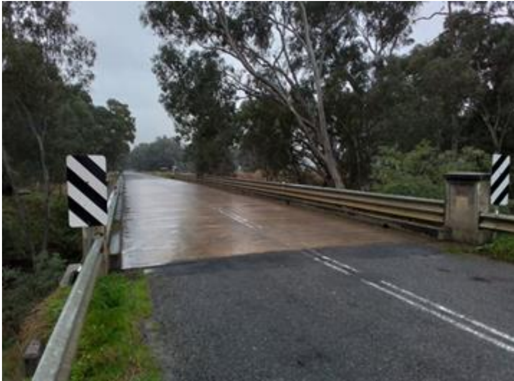
Billabong Creek Bridge – built in 1937
