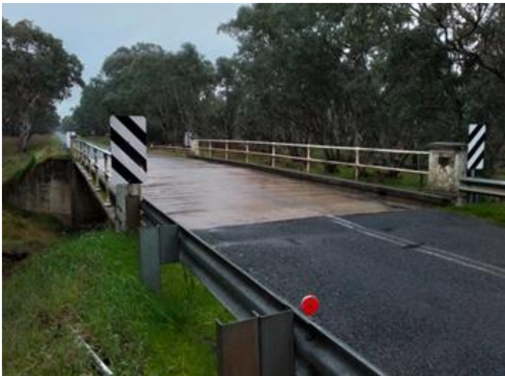
Back Creek Bridge – built in 1935
