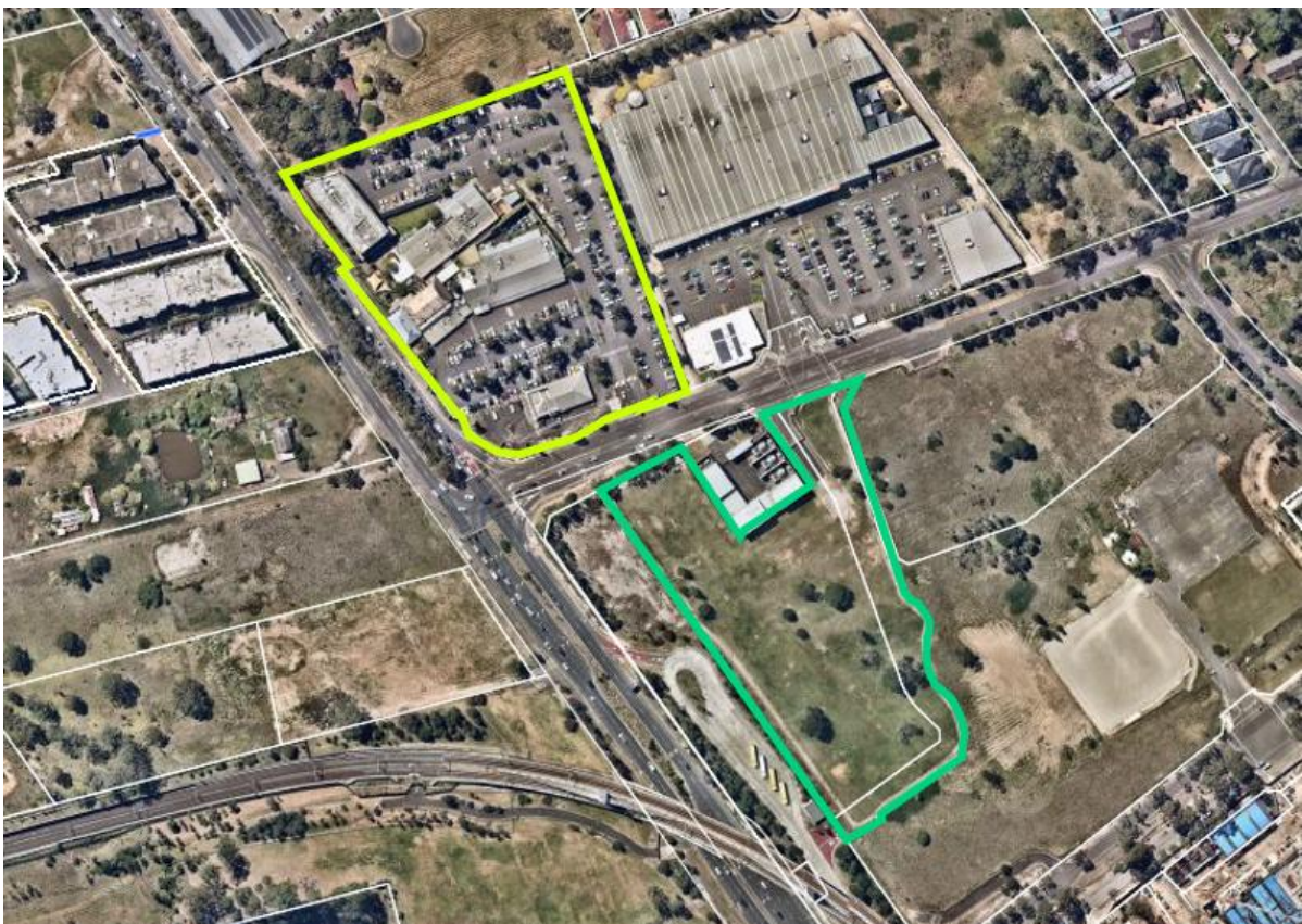
Figure 1: An aerial photo of the proposed hospital site (green border) and our client's site (yellow border). Image source: Mecone Mosaic
