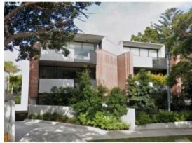
Picture 3 – RFB at 1 Spencer Street to the south
