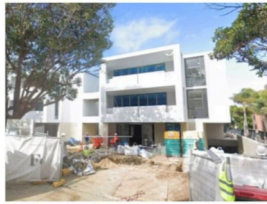
Picture 4 – RFB under construction at to the south
