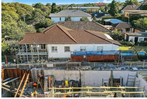
The front rooms of a house next to a development site on Wilberforce Avenue in Rose Bay caved after the excavation of a single storey. Ray White
