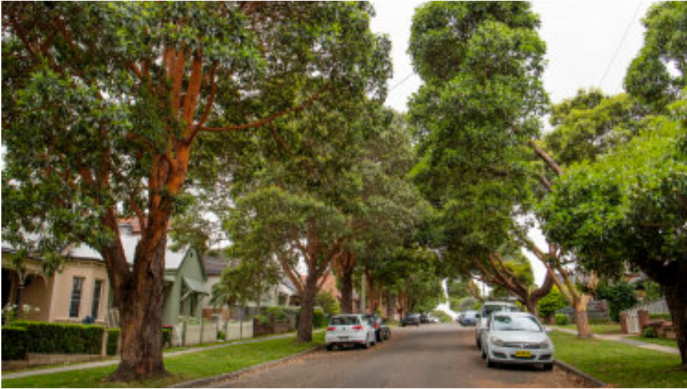
2. CARRINGTON STREET STRATHFIELD HOMES WHERE DAMAGE IN FOLLOWING THREE PHOTOS OCCURRED DURING TUNNELLING .
