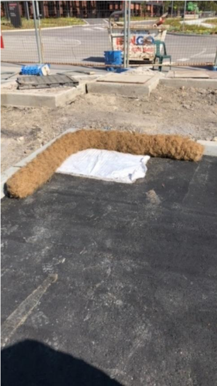
Figure 5: implemented sediment controls – northern carpark
