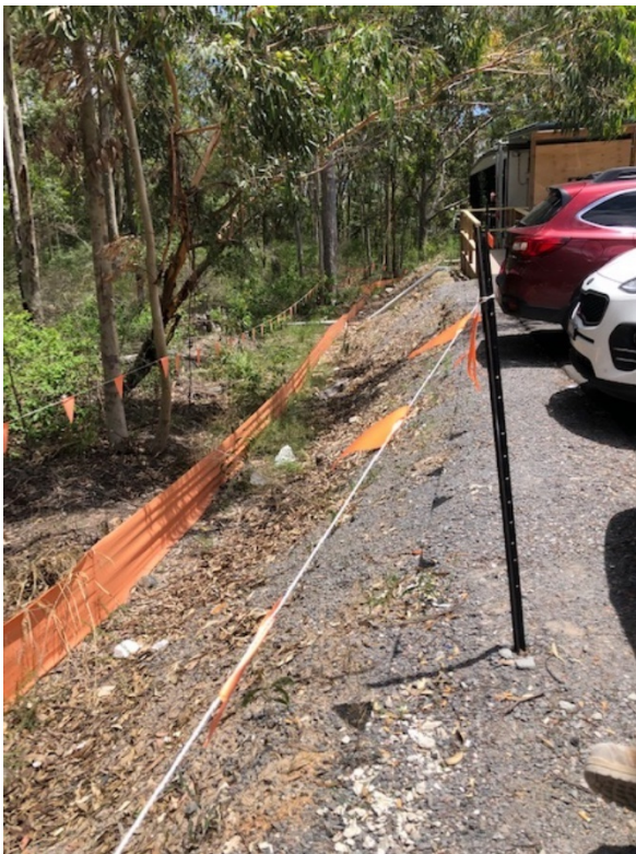
Figure 3: Showing Sediment controls at boundary and tree protection zone
