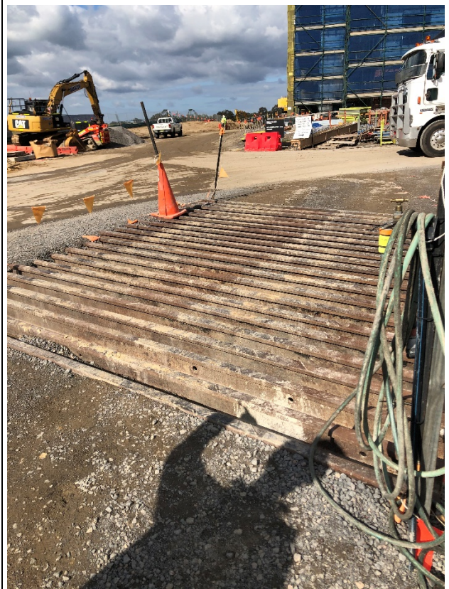
Figure 2: Showing rumble grid to prevent mud tracking
