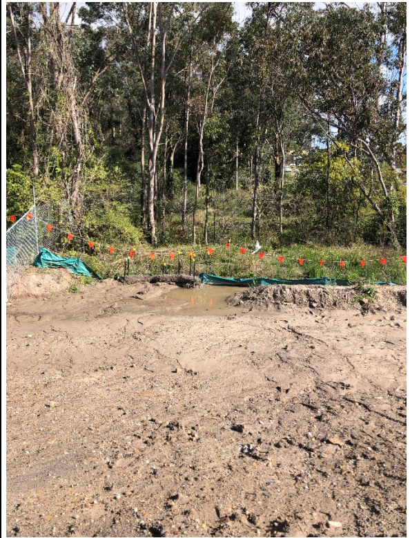
Figure 6: At capacity sediment controls, boggy ground and site delineation
