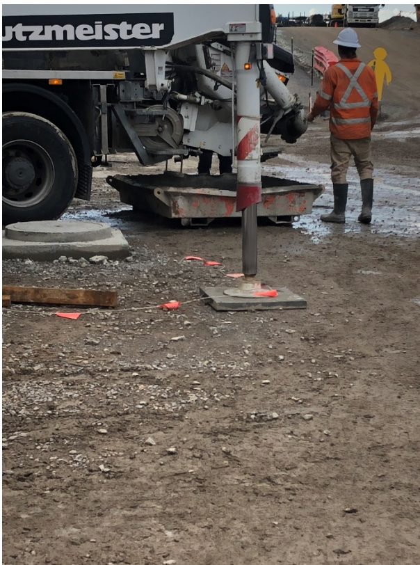
Figure 1: Showing concrete washout
