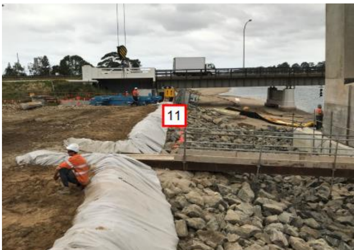
11) Keep silt curtains in place while detailing the permeant rock scour. Ensure the upper bank has a 300mm high geo wrapped edge bund installed for erosion and sediment control.
