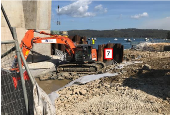
7) Install the working rock platform to project specifications.
