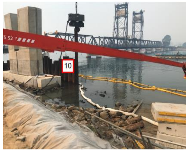
10) Keep maintaining the silt curtains during the works to ensure the curtains are secure and have the separation. Remove the coffer dams with vibrating hammer with Panolin oils only.
