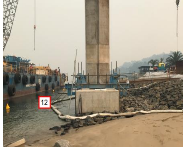
12) Remove the silt curtains from the river / canal. Remove the hydrocarbon boom and remove the buoys and anchors.
