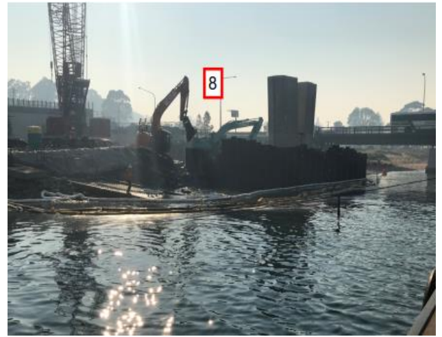
8) On completion of the structures work, remove rock platform. Install the permanent scour rock and permeant bank stabilisation.
