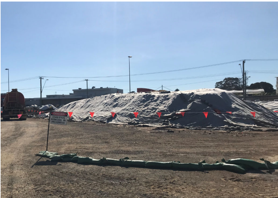
Figure 2 - Asbestos stockpile (Unexpected find)
