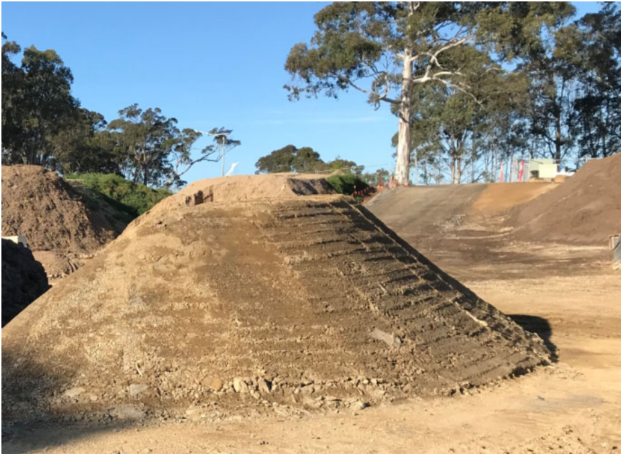
Figure 1 - Bucket pressed stockpile
