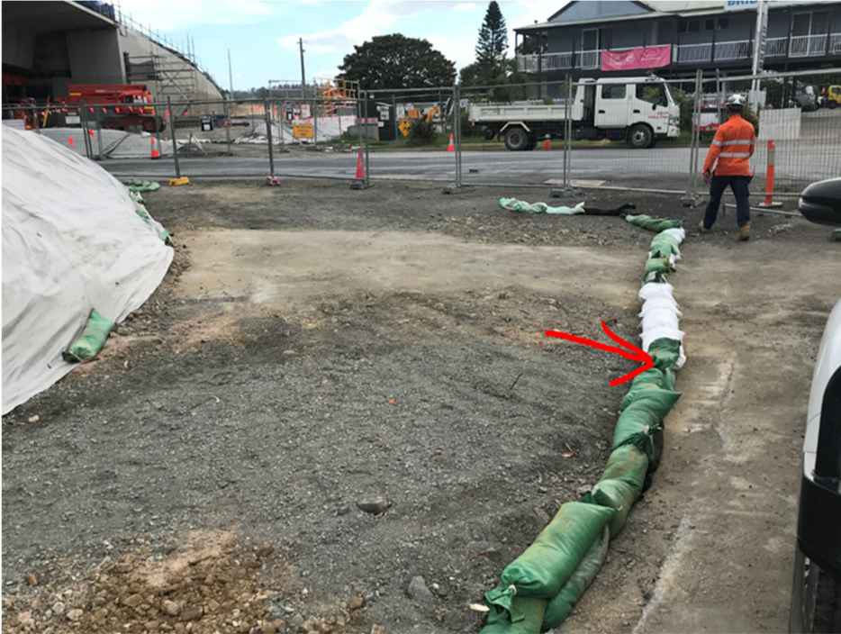
Figure 7 - Sandbag Controls
