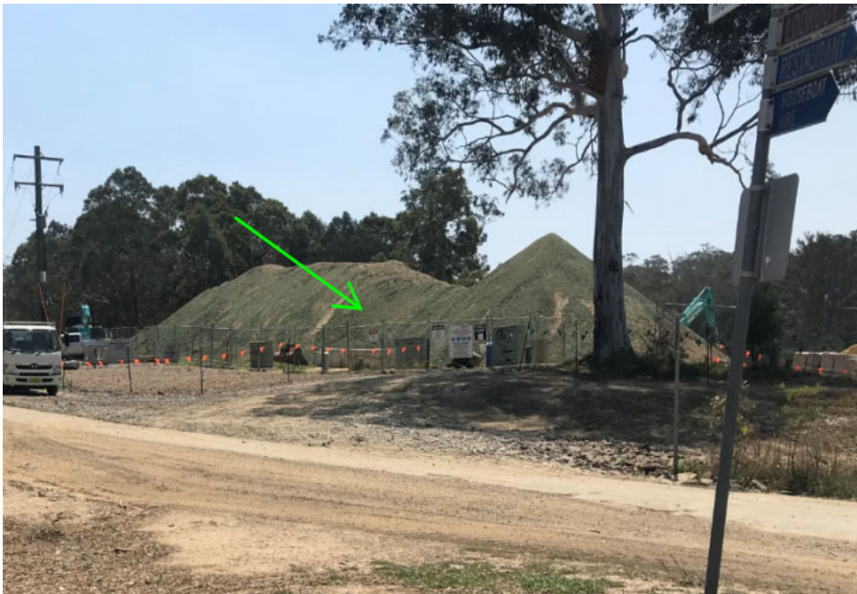
Figure 8 - Soil Binder Application
