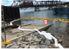
5) This photo demonstrates the disturb sediments settle back in the approved 'zone of disturbance'. This method ensures sediment does not migrate into the wider river / canal water column or surrounding ecosystems.
