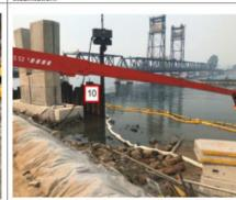
10) Keep maintaining the silt curtains during the works to ensure the curtains are secure and have the separation. Remove the coffer dams with vibrating hammer with Panolin oils only.
