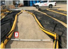
Manufacture the silt curtain separators from Erwin Clamps and strong aluminium conduit or similar. Test the curtain separator system before deployment of the floating silt curtains.
