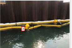
Prior to the install of the Coffer Dam. Install the double floating silt curtains, tie them off to the buoys and install separators. Install Hydro carbon boom on the inside of the curtains.
