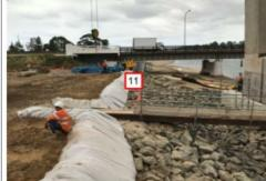
Keep silt curtains in place while detailing the permeant rock scour. Ensure the upper bank has a 300mm high geo wrapped edge bund installed for erosion and sediment control.
