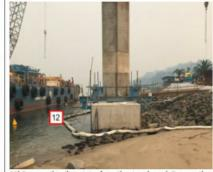
12) Remove the silt curtains from the river / canal. Remove the hydrocarbon boom and remove the buoys and anchors.
