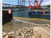
4) Installation and removal of the Coffer Dam will create sedimentation. This sedimentation occurs in the approved 'zone of disturbance'. If sedimentation occurs between the silt curtains gaps the works is stopped to allow settlement.
