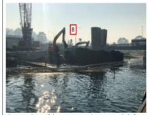
On completion of the structures work, remove rock platform install the permanent scour rock and permeant bank stabilisation.
