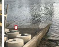
2) The floating silt curtains require buoys, chains and anchors. Ensure that the install of the anchors is conducted with a crane or a boat with a Hiab. Place the anchors gently on the river / canal bed to limit sediment disturbance.
