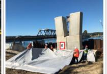
6) Once the Coffer Dams are installed and whaler beams fixed. Geotextile can be laid out inside the coffer dam to allow placement of the working platform.
