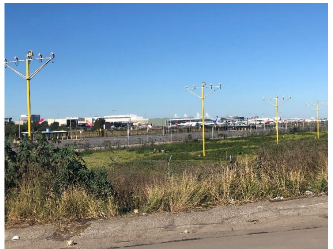
Figure 19.8 High intensity approach lighting
