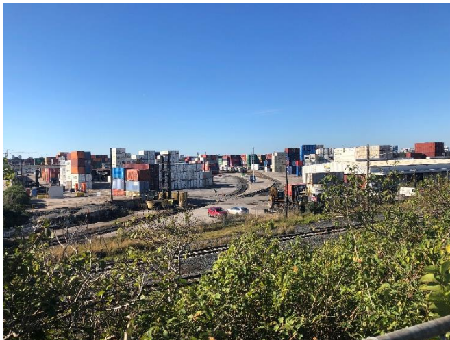
Figure 19.9 Cooks River Intermodal Terminal
