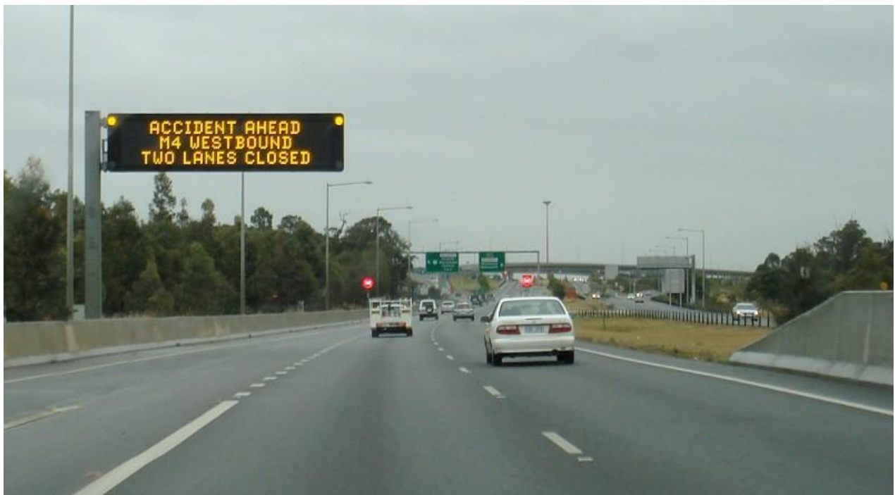
Figure 7.27 Typical variable message sign
