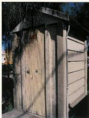
Figure 6-13 Precast concrete hut #1. Source. NSW OEH
