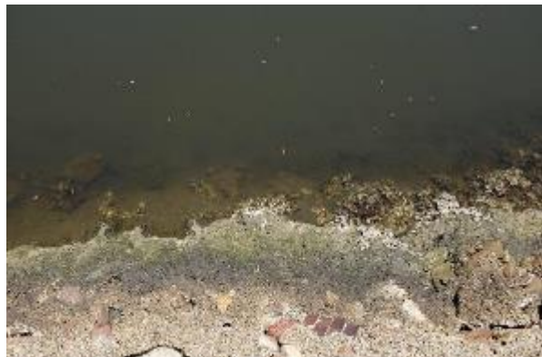
Figure 13-45 Detail of modern Alexandra Canal retaining wall along south side of the canal. Note modern brick used as aggregate during construction.
