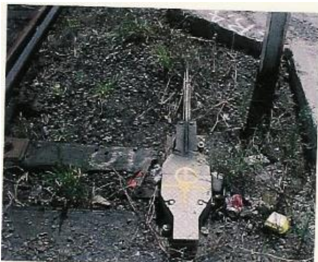
Figure 6-12 The spiked down modified Thompson lay down points lever at Road 7. Source. NSW OEH
