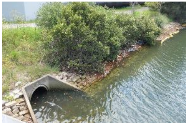
Figure 13-43 Detail of modern culvert installed along west bank of the Alexandra Canal between original sandstone wall. Taken from pedestrian footbridge, facing north.
