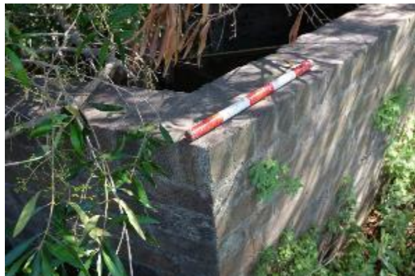
Figure 13-62 Detail of brick weir/water management structure (0.5 metre scale).
