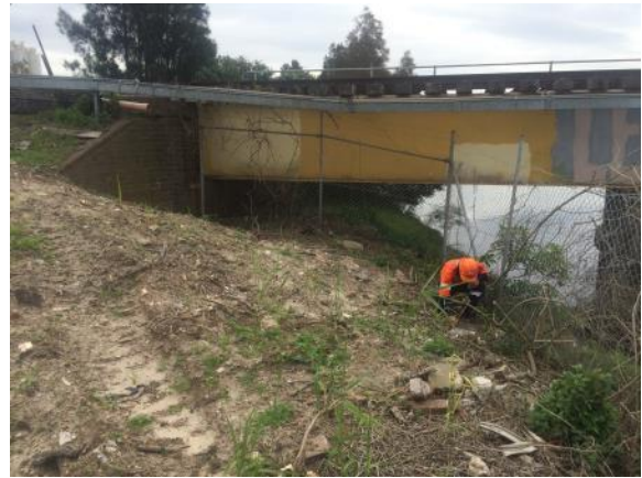
Plate 8. Survey Unit 3 facing east showing bank constructed from redeposited sandy fill with modern inclusions corridor
