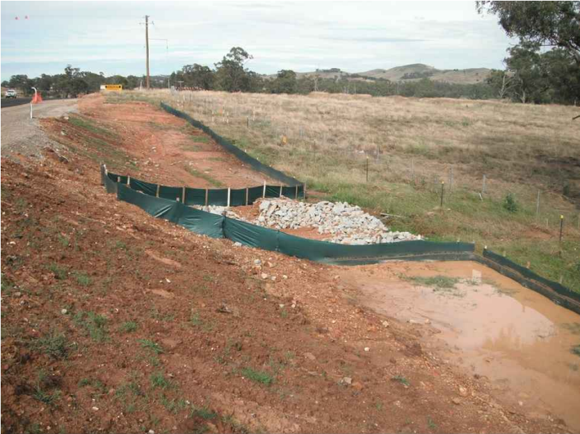
PHOTO 1: EXAMPLE OF SILT FENCE WRAPPED UP AND BEHIND PIPE OUTLET.
