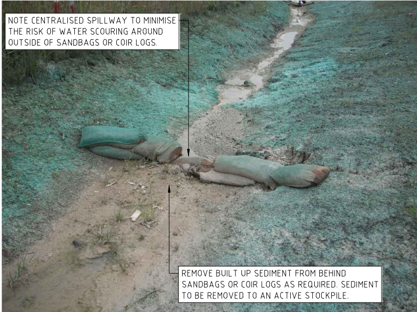
PHOTO 2: EXAMPLE OF CHECK DAM WITH CENTRALISED SPILLWAY.
