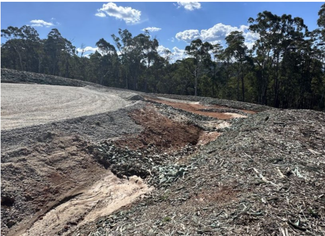
Plate 24: Rock drains located along the western alignment (Inspection Date: 12/03/2025).
